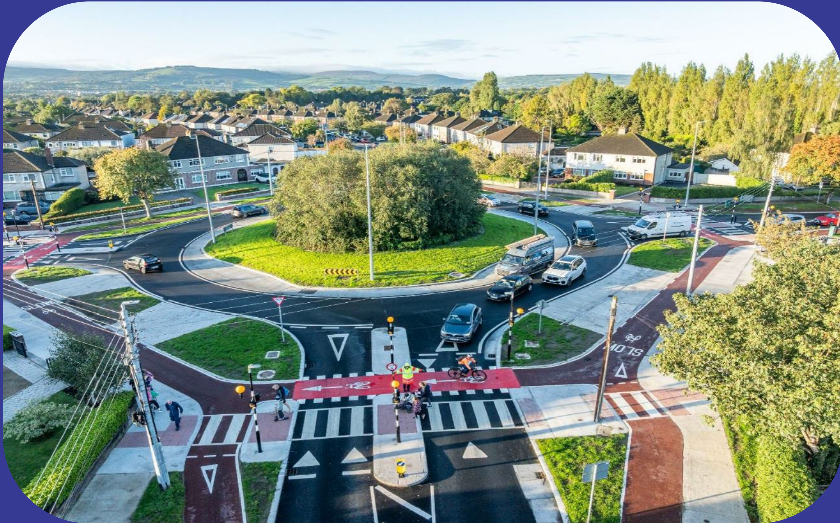
Aerial view of upgraded Templeville / Wainsfort Roundabout
