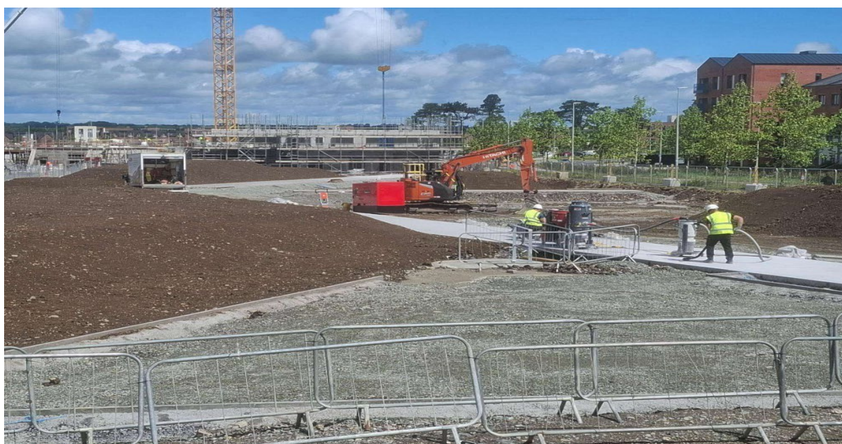
Works on Central Boulevard Park in Adamstown
