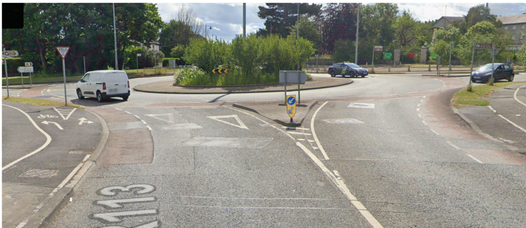
Figure 5: Ballyboden Road / Taylor's Lane Roundabout, multi-lane approach with no safe crossing
