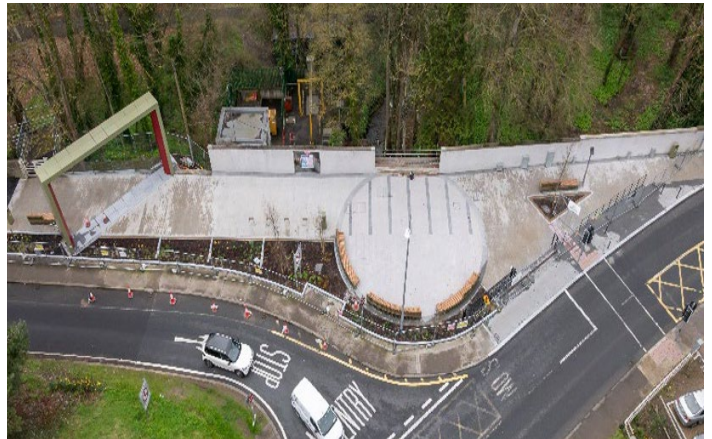
Aerial views of works at Lucan Village (top) & Lucan Demesne (bottom)
