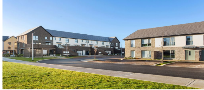
New affordable homes at Keepers Lock
