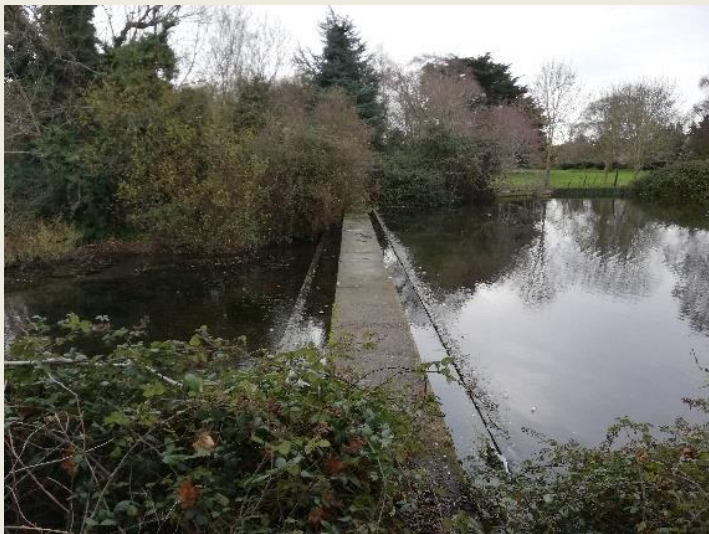
3) Mill pond south of Clondalkin Leisure Centre, which now occupies the former mill race.
