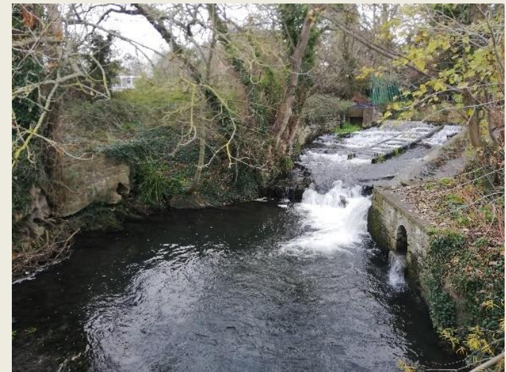
1) Historic weir (Reg. no. 11209042) associated with the Mill Race and pond. There is a large scour pool at the downstream end.
