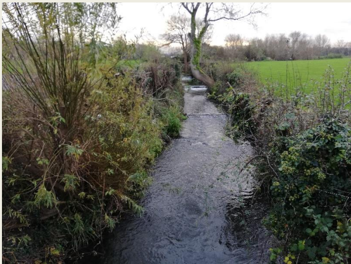
2) Looking US: Channel is realigned, with 2 weirs seen in the distance. The riparian zone is very narrow, with manicured grass on both banks.
