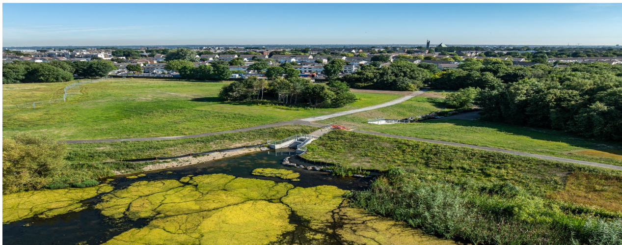
• Embankment and flow control structure at Tymon Park Lake
