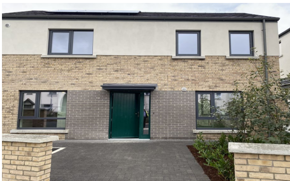
Recently completed home at Watercourse Grove
