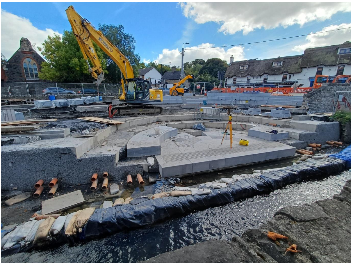
Figure 1 progress in the main amphitheatre in the Village Green. note main masonry blocks are being positioned.
