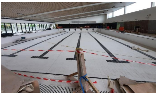
Pool tiling completions, cleaning, and finishing work ongoing
