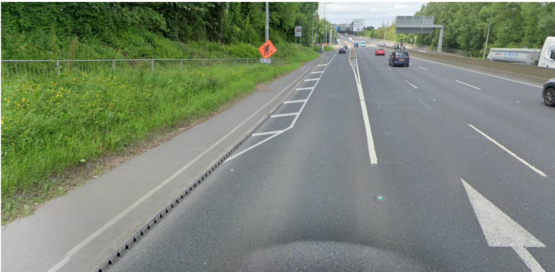
View of approach towards the N4J4a slip lane from the motorway, illustrating proposed hatch markings to narrow lane widths
