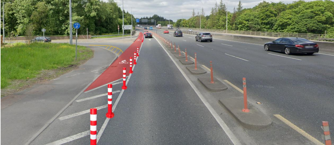
View of approach towards the L1018 junction from the slip lane, illustrating proposed bollards and red surface treatment to existing cycle lane.
