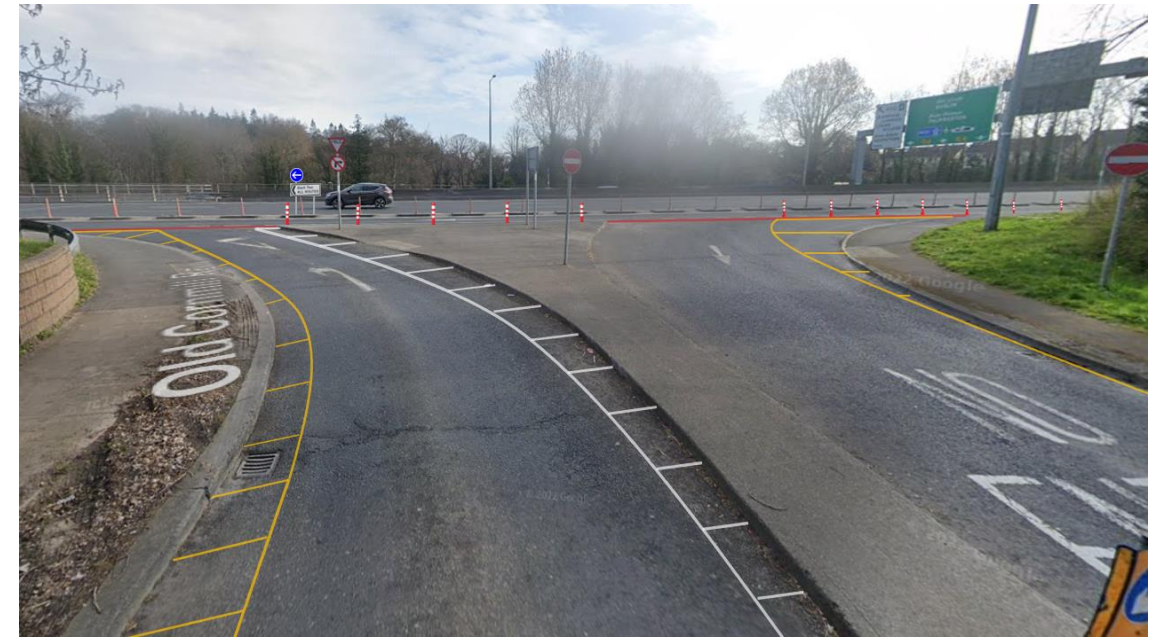
View of approach towards the N4J4a slip road from the L1018 Junction, illustrating additional road markings and bollards.
