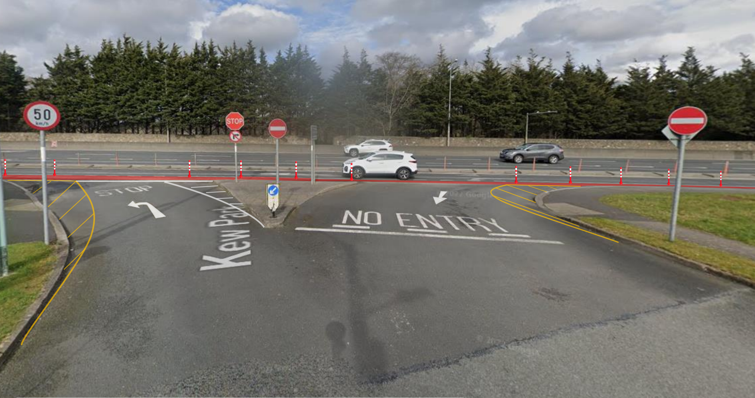
View of approach towards the N4J4a slip road from the Kew Park Junction, illustrating additional road markings and bollards.
