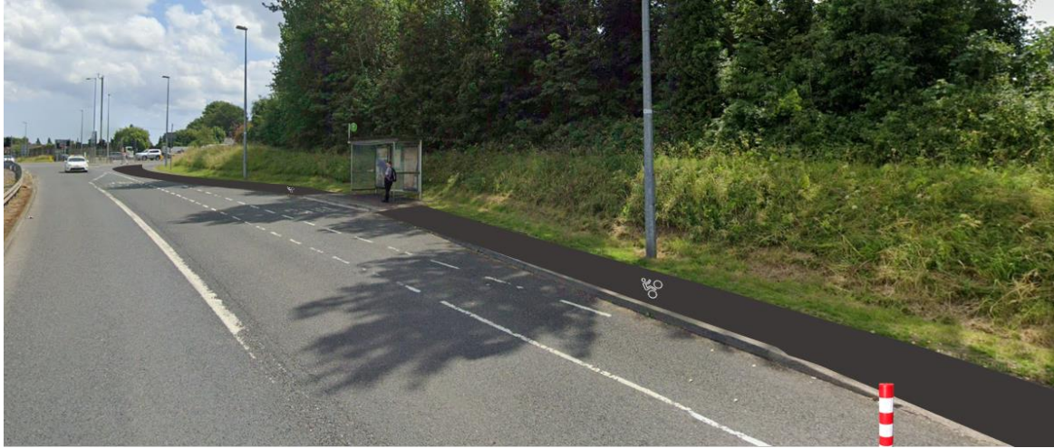
View of Leg 2 bus stop with cycle track and shared space link
