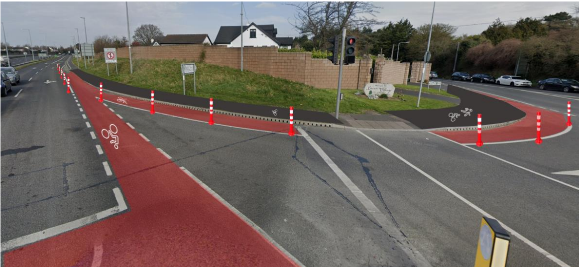
View of Leg 3 with proposed bollards and restoration of red surfacing
