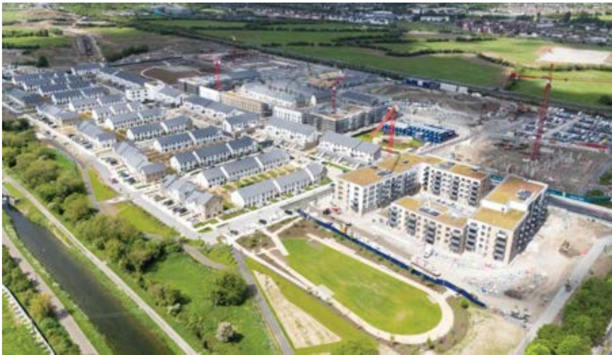
Clonburris SDZ – Current build out of residential units at Clonburris SDZ.
