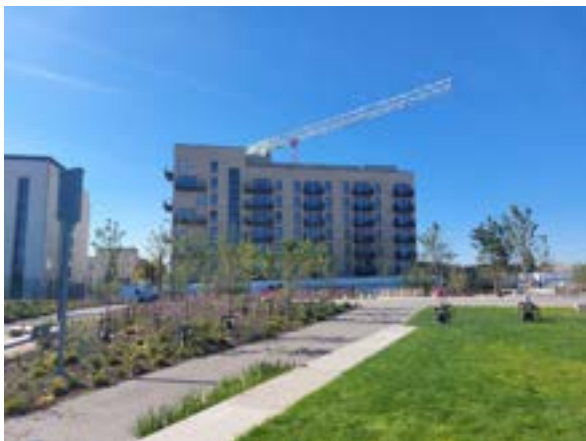
Belgard Square North – the first Council led cost rental scheme which will also be served by the Tallaght District Heating Scheme
