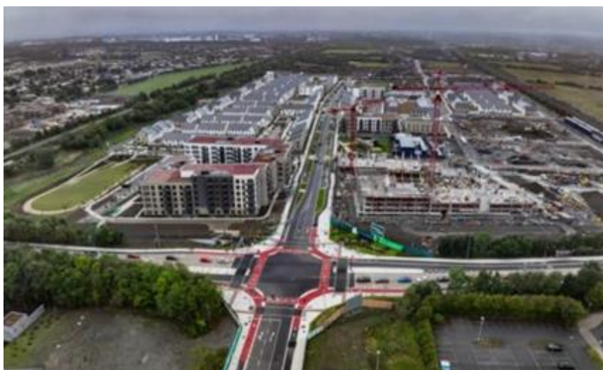
Clonburris SDZ – Progress on the build out of the Southern Link Street and housing, south of
