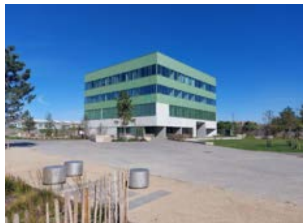
New Innovation Centre in Tallaght Town Centre
