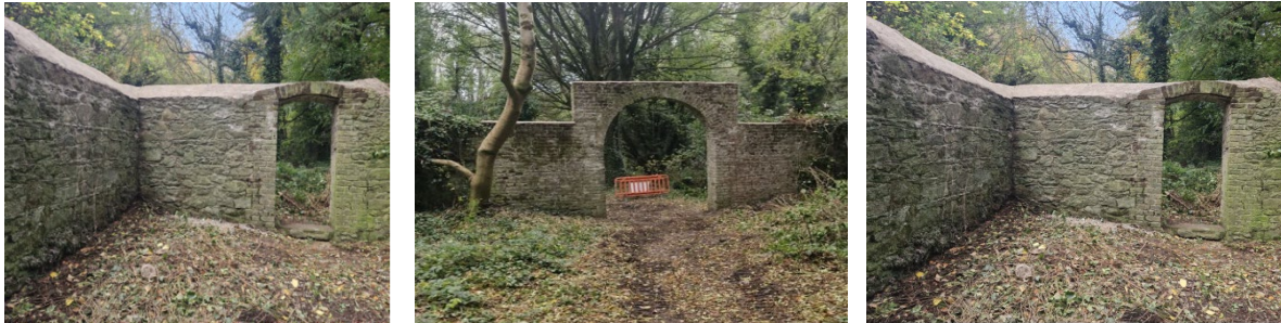
Conservation Works at Massy's Woods
