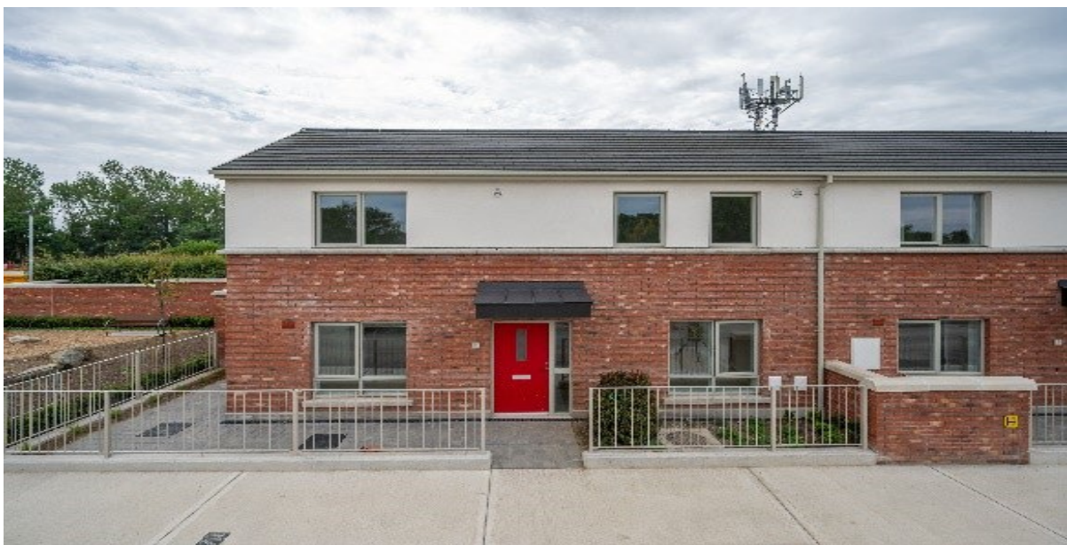
Completed Development of Social Homes at New Nangor Road
