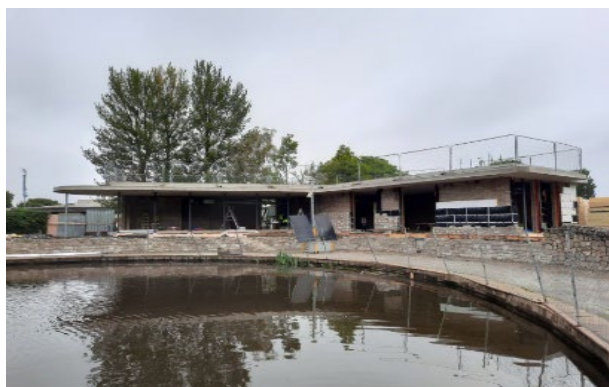
Works progressing at Tymon Intergenerational Centre
