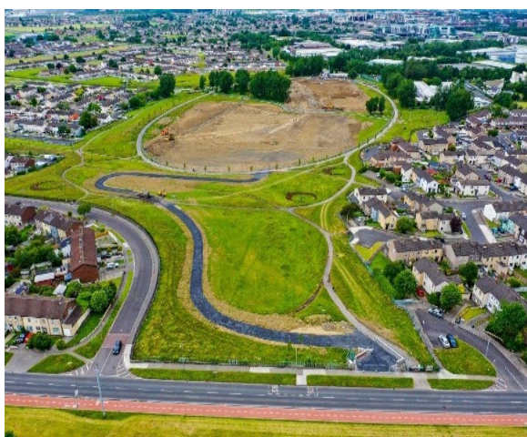
Aerial view of works at Killinarden Park
