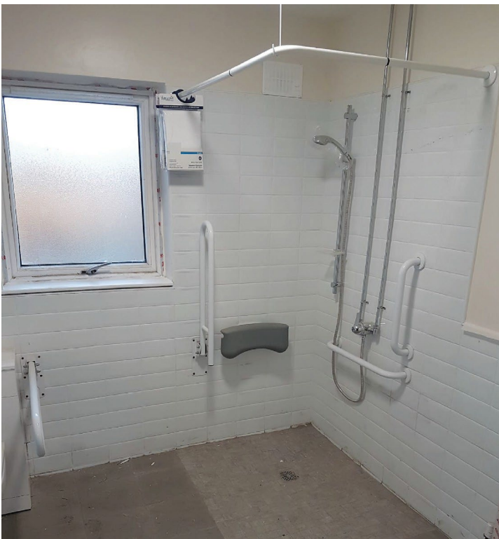
Level Access shower installed in a local authority home
