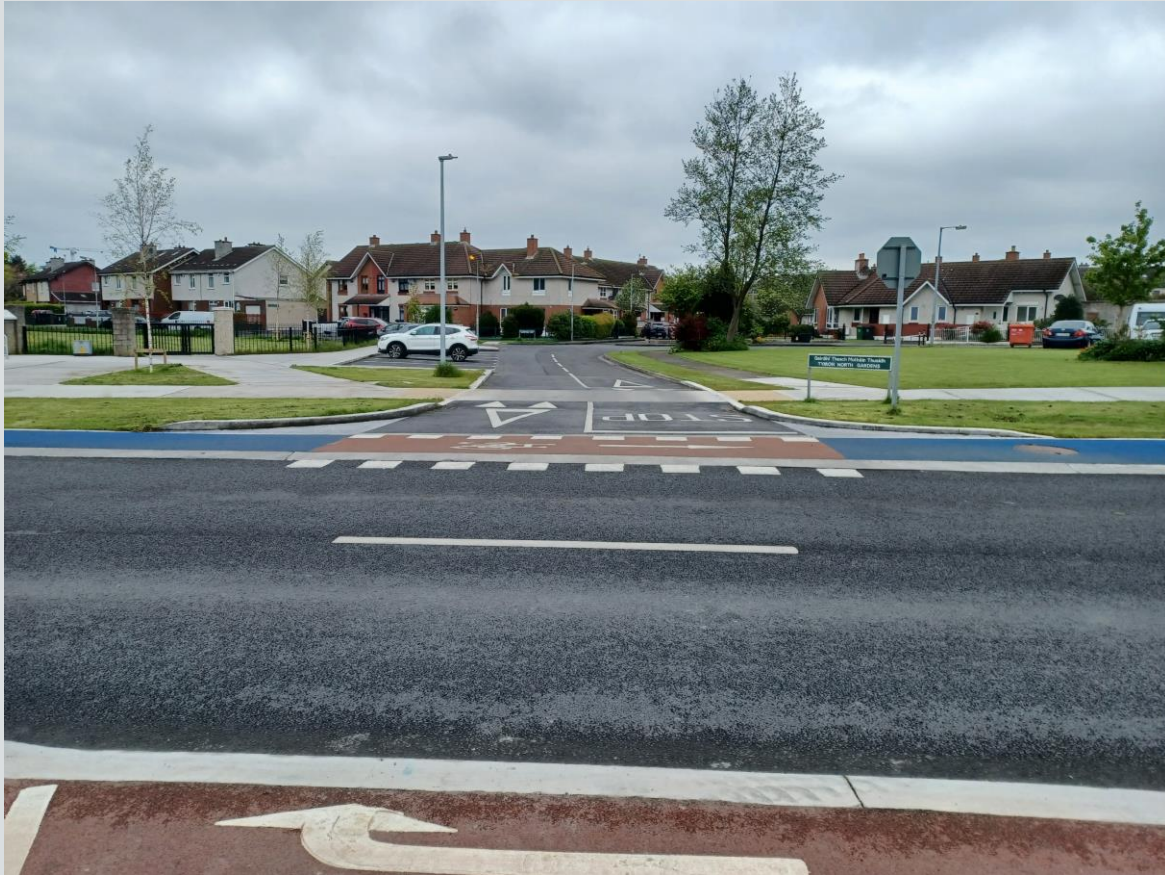
District Centre Enhancement
