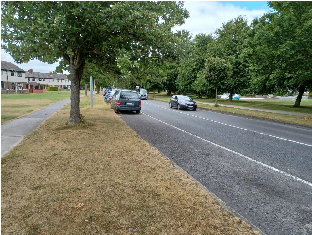
Figure 1-3: Existing Castletymon Road South
