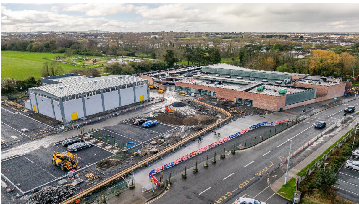
Aerial view of works at Lucan Leisure Campus
