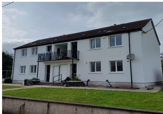
Completed EERP Works at St. Maelruan's Park
