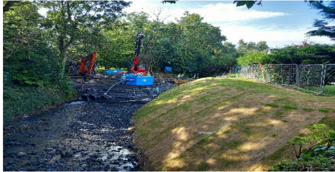
Whitechurch Flood Alleviation Scheme Works are ongoing
