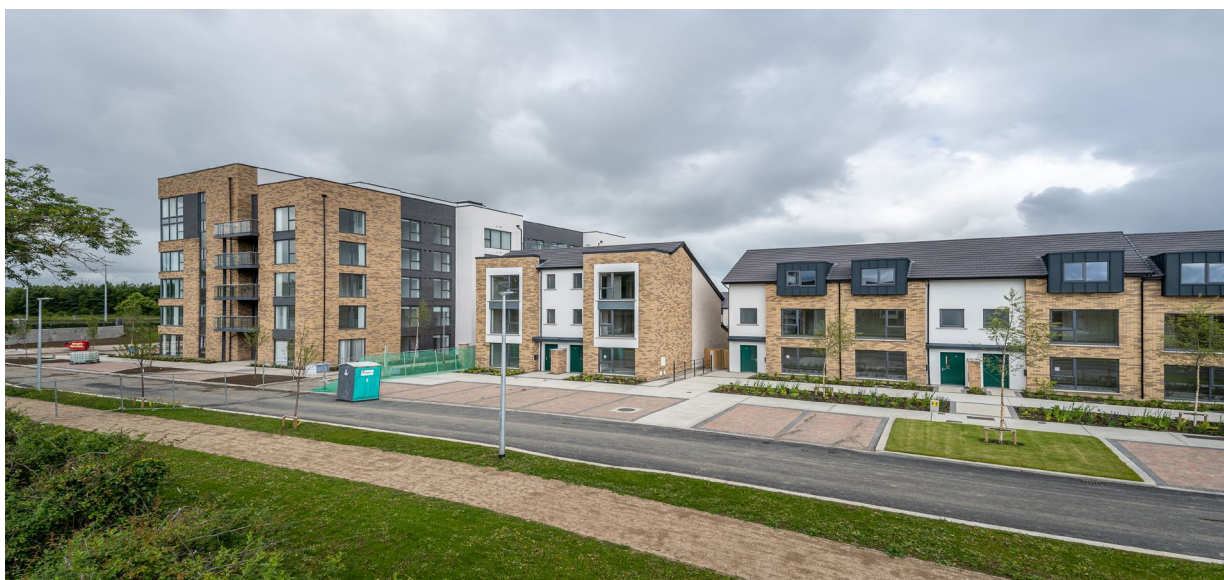
Delivery of social and affordable housing continues at Kilcarbery Grange
