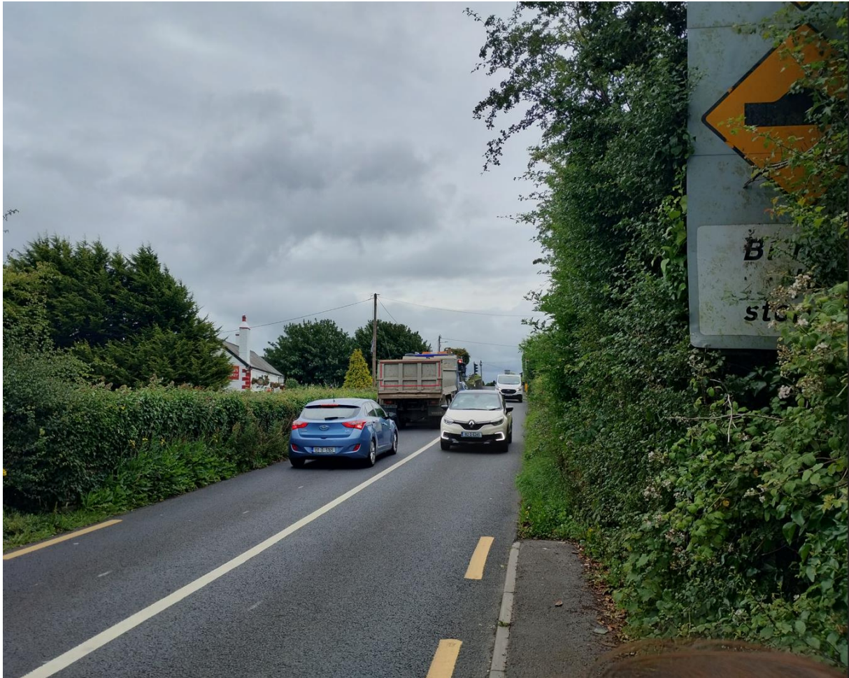
Figure 6: Existing footpath north of the bridge on western side of carriageway showing overgrown vegetation obstructing signage (Photo taken July 2023)
