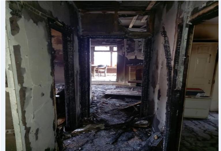
**Figure 15-8: Fire Door protection to room after fire**
