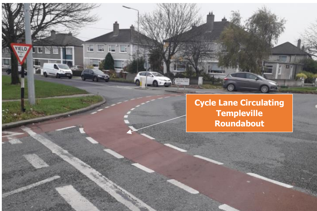
Figure 3-12: Cycle Lane at the Templeville Roundabout
