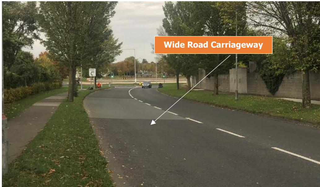
Figure 3-3: Wellington Lane road carriageway on approach to Orwell Roundabout
