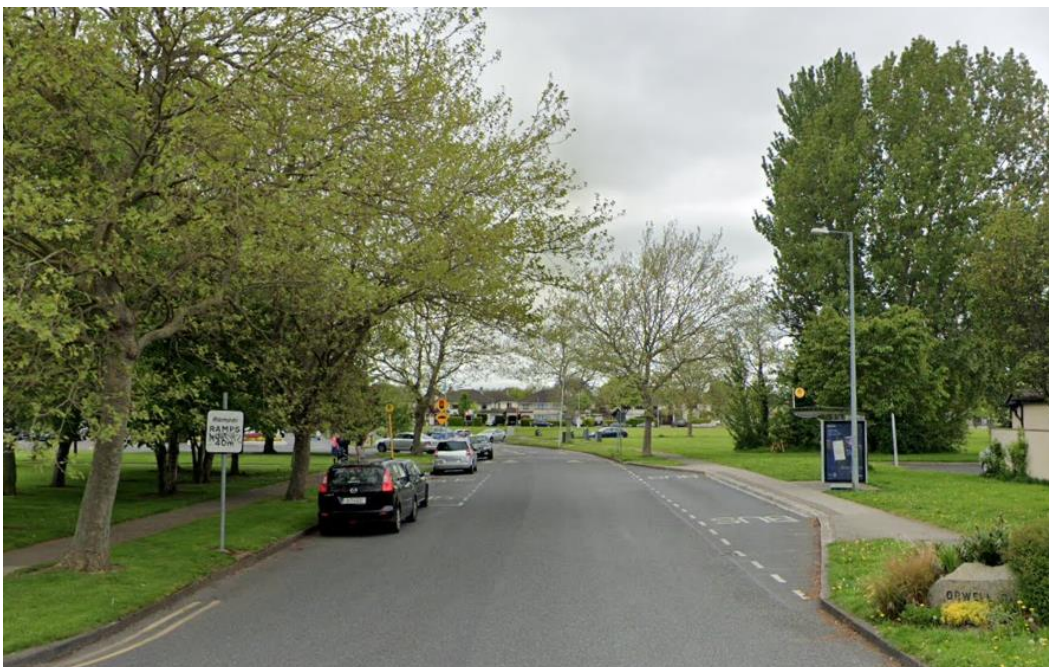
Figure 3-19: Existing Road Carriageway at Orwell Road
