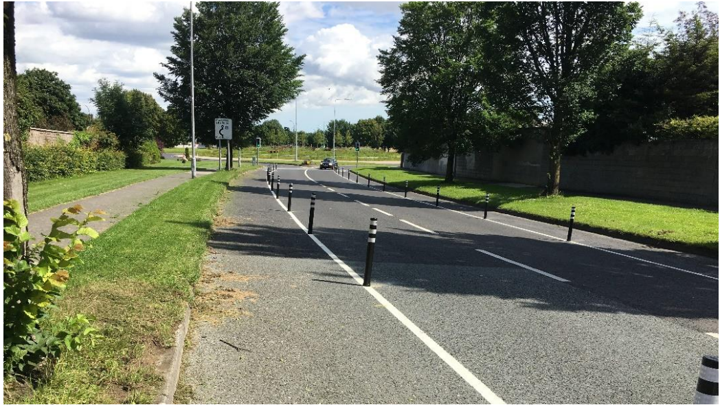
Figure 3-6: Current protected on road cycle lanes on approach to Orwell Roundabout
