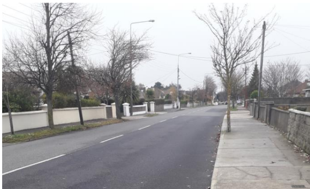
Figure 3-16: Whitehall Road Carriageway
