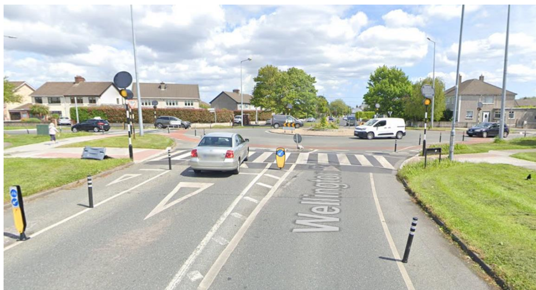
Figure 3-14: Temporary zebra crossings at Templeville Roundabout (Source: Google Maps)
