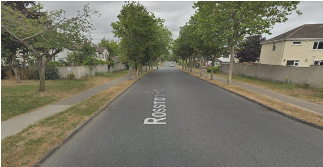
Figure 3-18: Existing Road Carriageway at Rossmore Road
