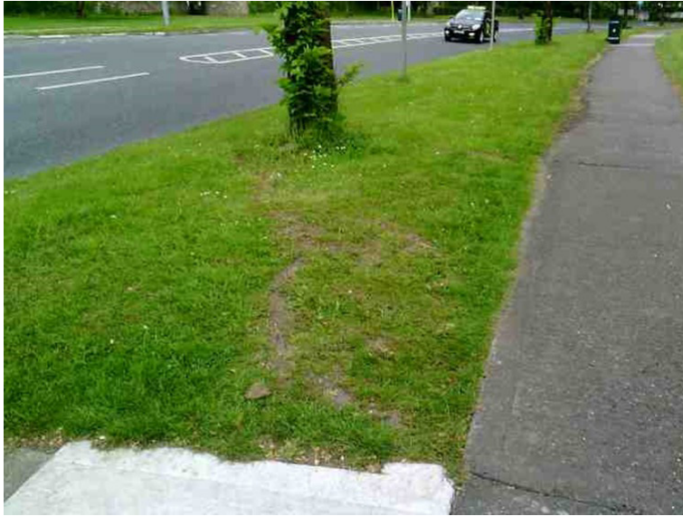
Image 33. Mower impact damage to surface roots of elm within grass verge on Wellington Lane. Note repair work to paving at base on image.
