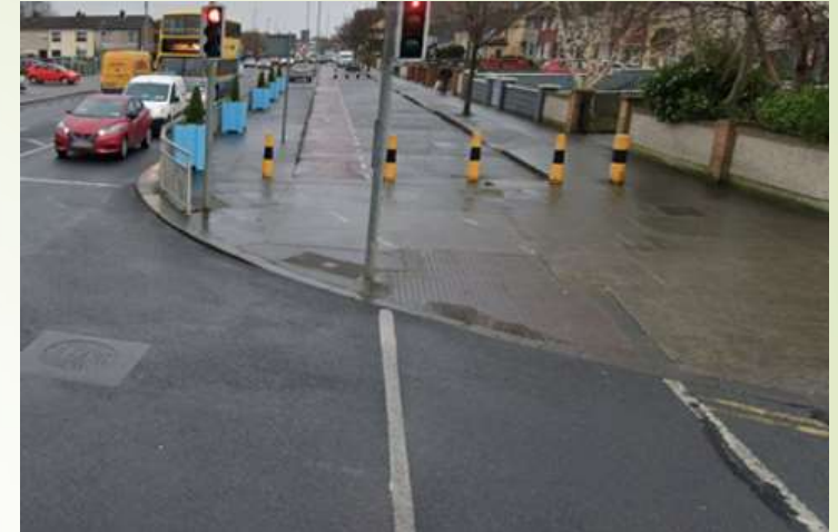
Level 2 - Cyclists share pedestrian crossing and give way to side road traffic.
