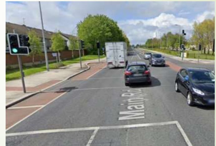
Level 4 - Provision suitable for a non-confident cyclist to safely make all movements. Cyclists do not share space with pedestrians.
