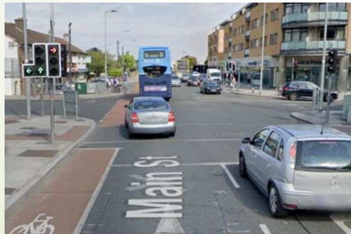
Level 3 - Provision for a non-confident cyclist to make a left and straight ahead movement. No provision for right turns without conflict
