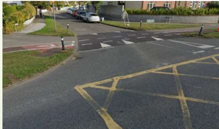
Level 3 - Cyclists have dedicated infrastructure to take them across side road separately to pedestrians, however it may be unclear who has priority between cyclists and cars
