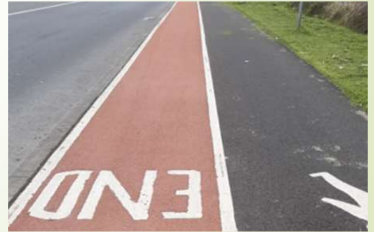
Level 4 - Good, no action required.
