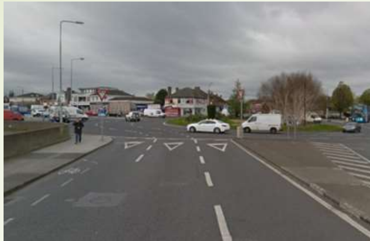
Level 1 - No cycle provision, or cycle provision stops short of junction. Multiple lanes to cross makes the junction dangerous even for confident cyclists.
