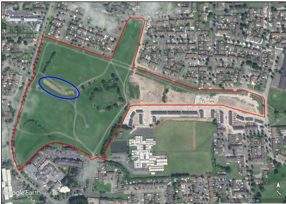
Figure 20: St. Cuthbert's Park aerial view, Google Earth, July 2019.
