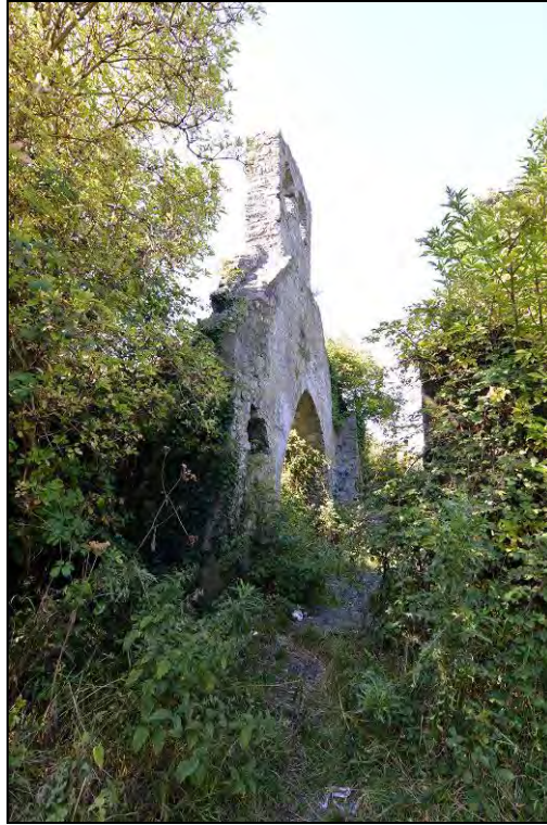
Photograph 9: Chancel arch and bellcote, viewed from the south.
