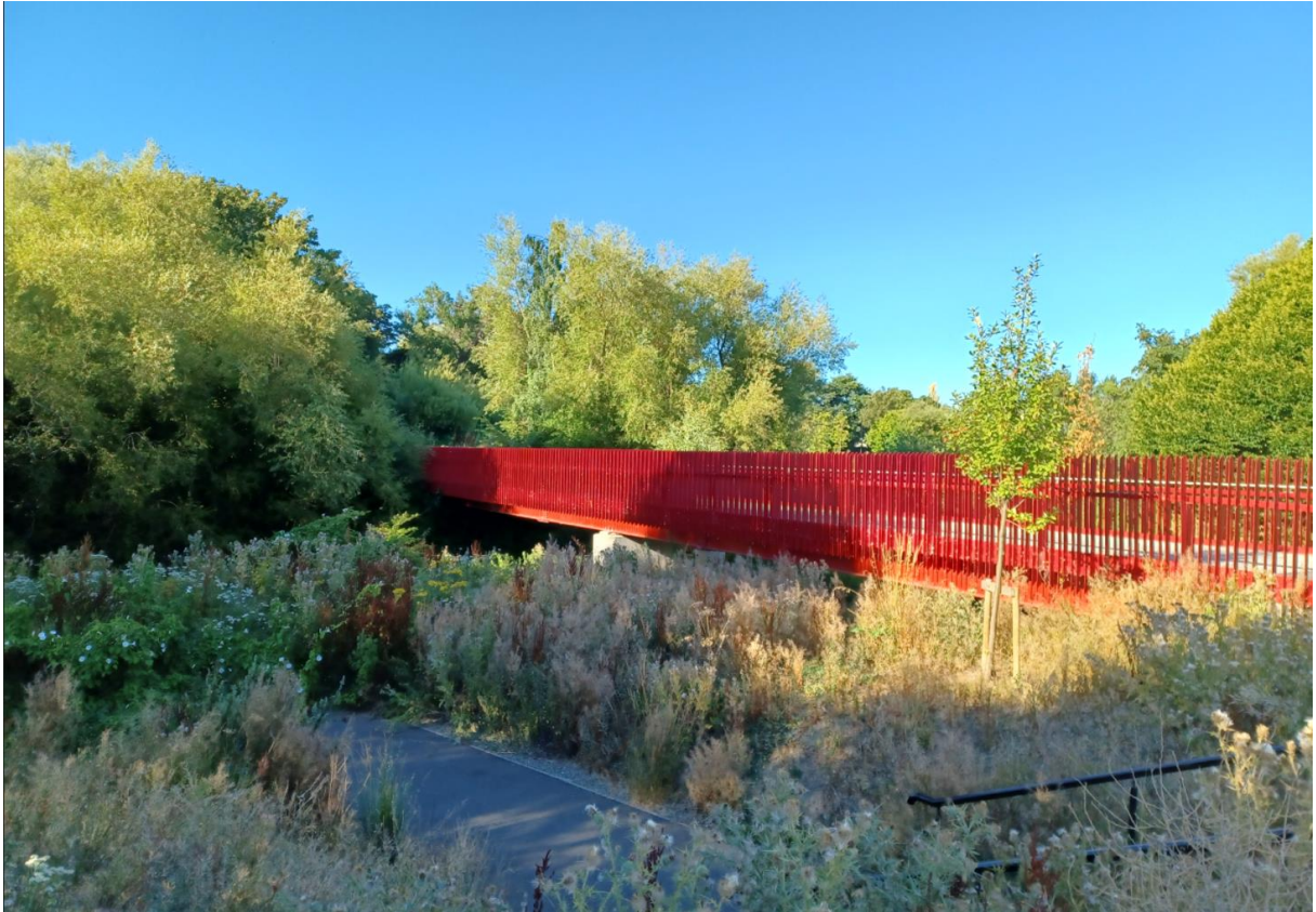
Figure 2-6: Proposed Bridge Design Precedent - Steel Through-Truss Arrangement Supported on Concrete Abutments (Source: Arup)
