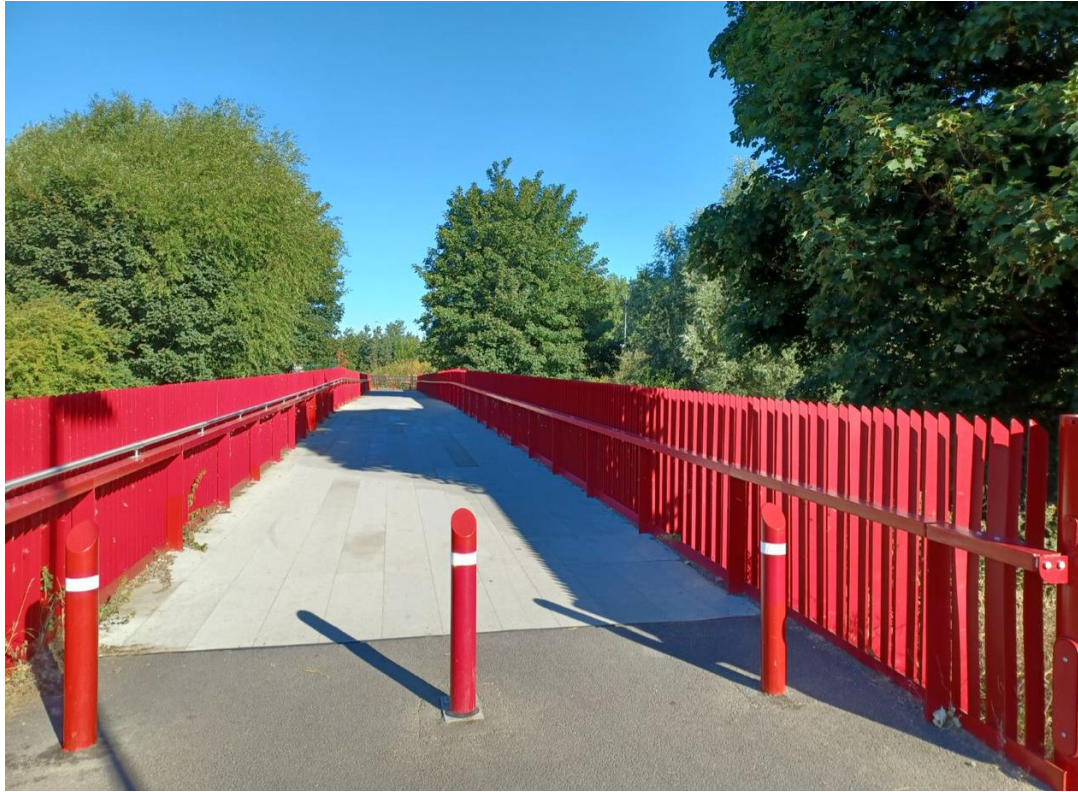
Figure 2-4: Proposed Bridge Design Precedent – 4m wide Shared Pedestrian and Cycle Connection (Source: Arup)
