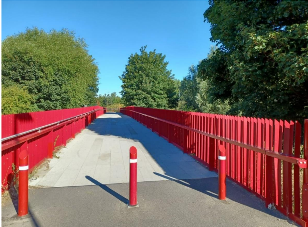
Figure 2-4: Proposed Bridge Design Precedent – 4m wide Shared Pedestrian and Cycle Connection (Source image: Arup)
