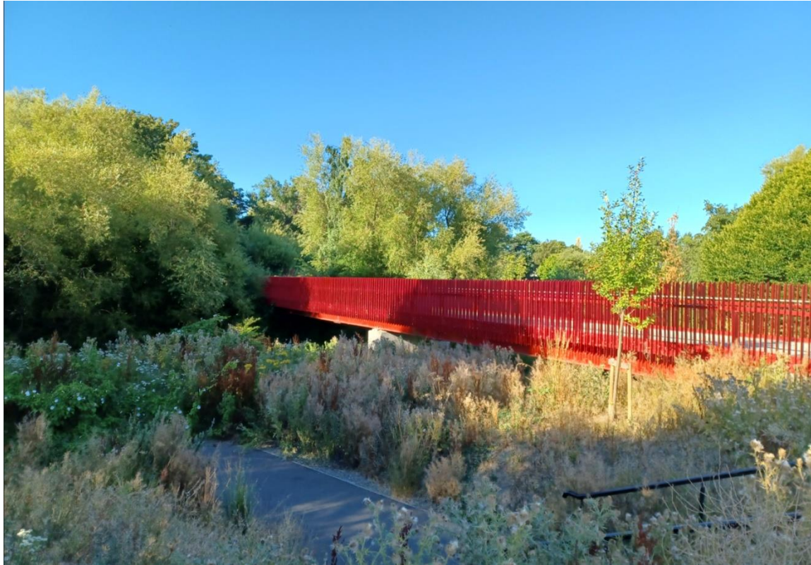
Figure 2-6: Proposed Bridge Design Precedent - Steel Through-Truss Arrangement Supported on Concrete Abutments (Source image: Arup)
