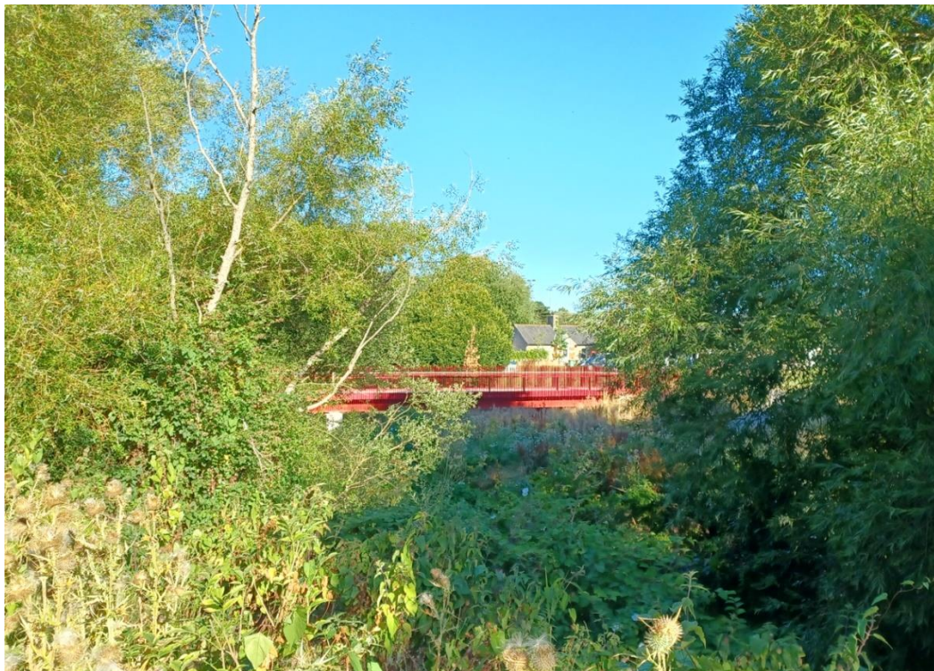
Figure 2-5: Proposed Bridge Design Precedent - Steel Through-Truss Arrangement Supported on Concrete Abutments (Source image: Arup)
