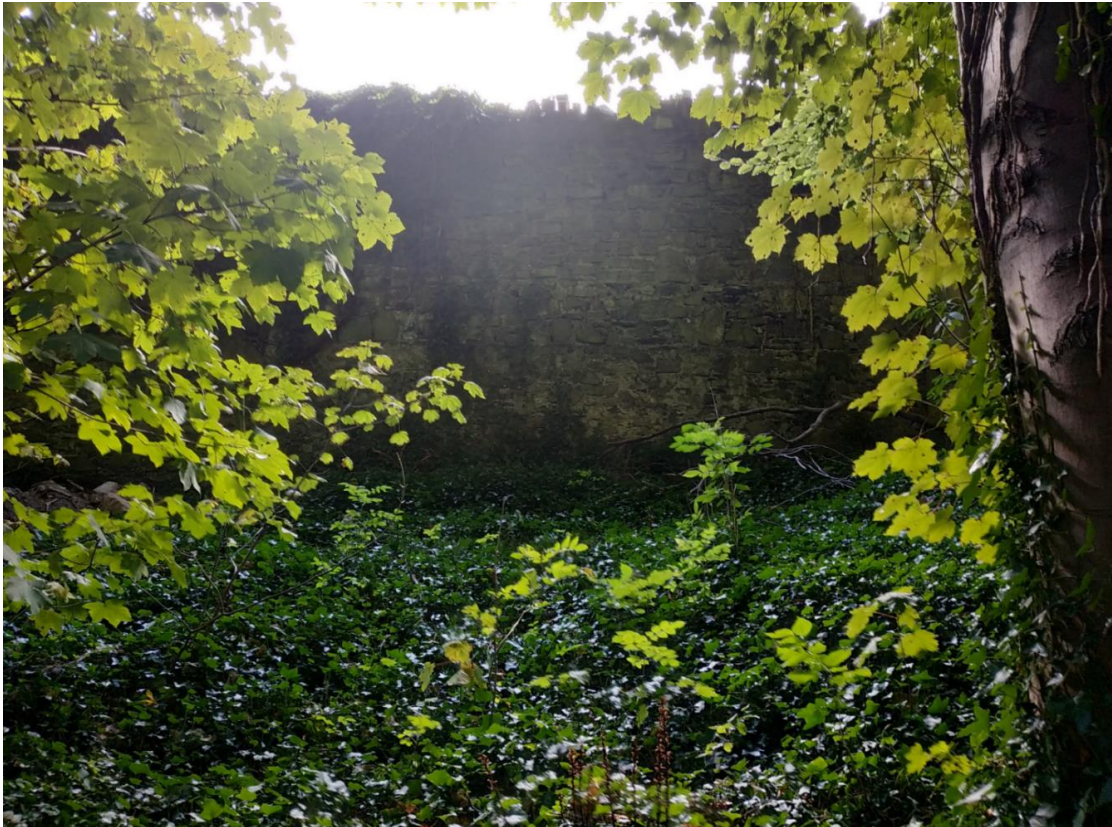
Photograph 4 Looking to the South. Remaining retaining wall section
