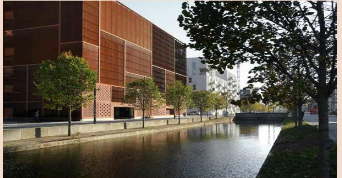
Figure 144. ParkingHus in Ørestad, street view
