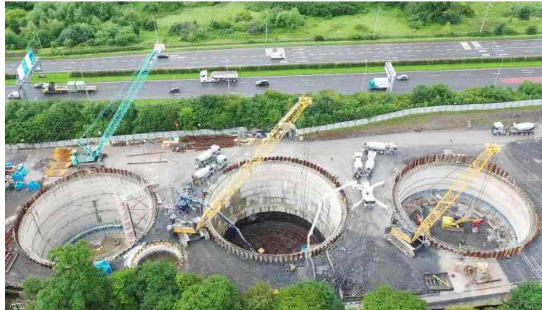
Figure 279. An aerial view of the 9C sewer upgrades in Blanchardstown (similar in scale to potential 9B upgrades) which included 3 no. shafts of a similar size. This provides an appreciation of the spatial requirements.
