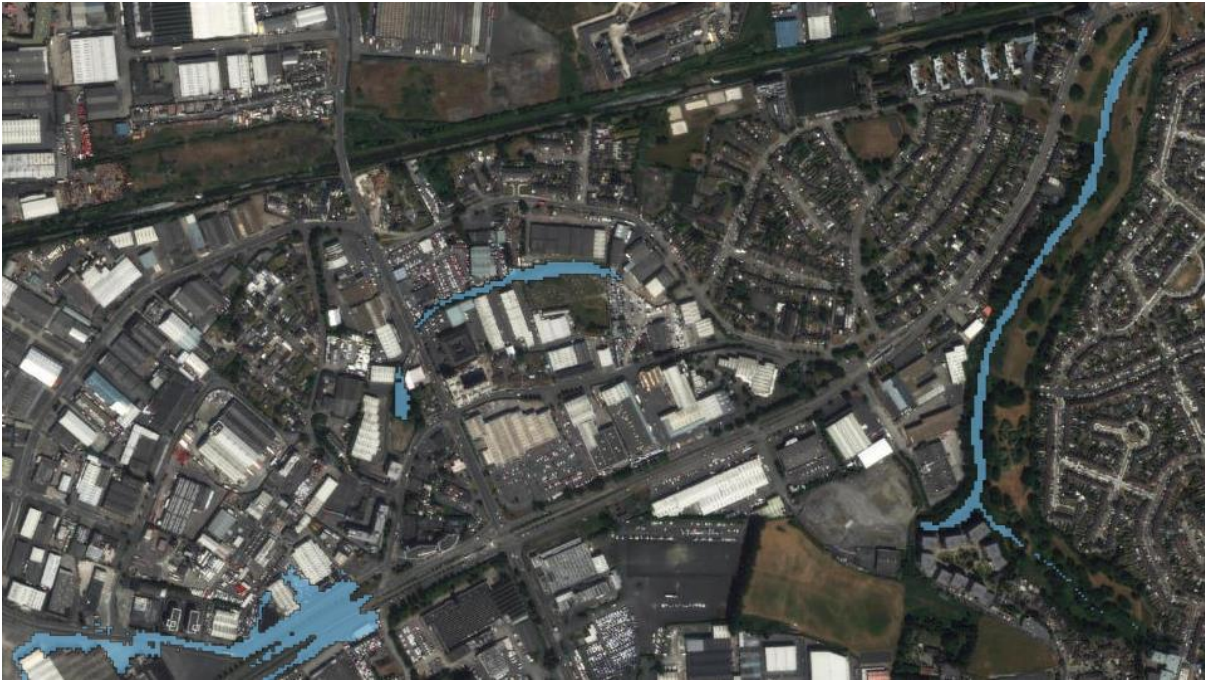
Figure 5-8: Flood Zone B – Naas Road and John F. Kennedy Drive
