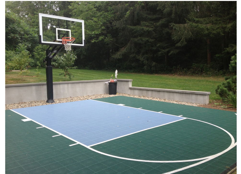
HALF BASKETBALL COURTS
