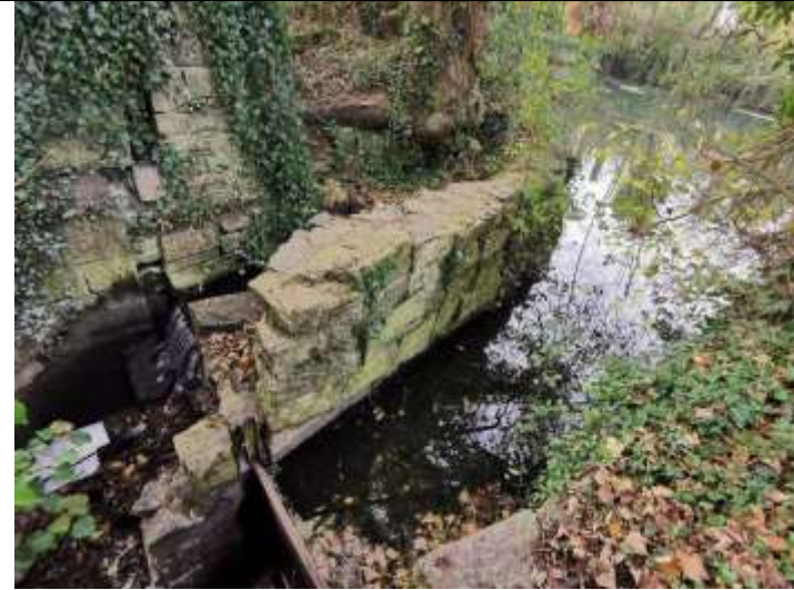
Plate 14 View of sluice, facing southeast
