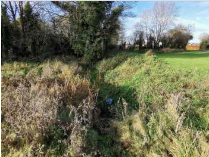
Plate 51 View of CH13, former tail race, facing west
