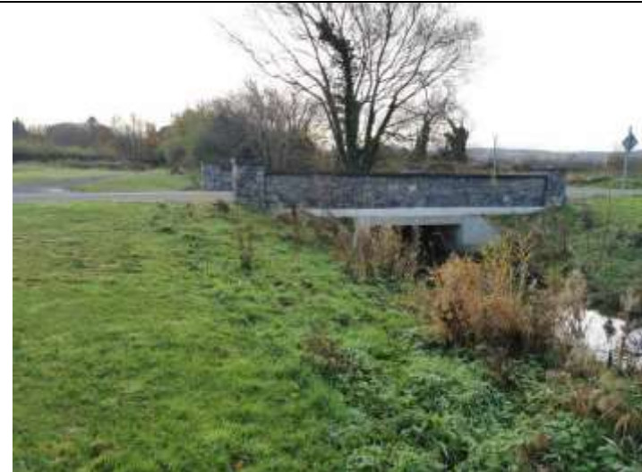
Plate 8 Modern access bridge over Camac River, facing southeast
