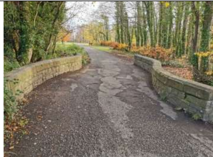
Plate 44 View of northern bridge, facing northeast
