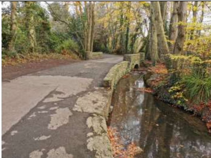
Plate 43 View of bridge, facing northeast
