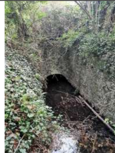
Plate 16 View of arch to culver to tailrace, facing east
