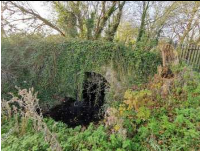
Plate 49 View of CH12 former bridge, facing south
