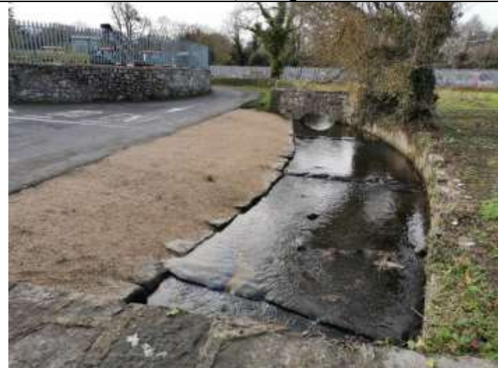
Plate 36 Northern curvilinear watercourse, facing west
