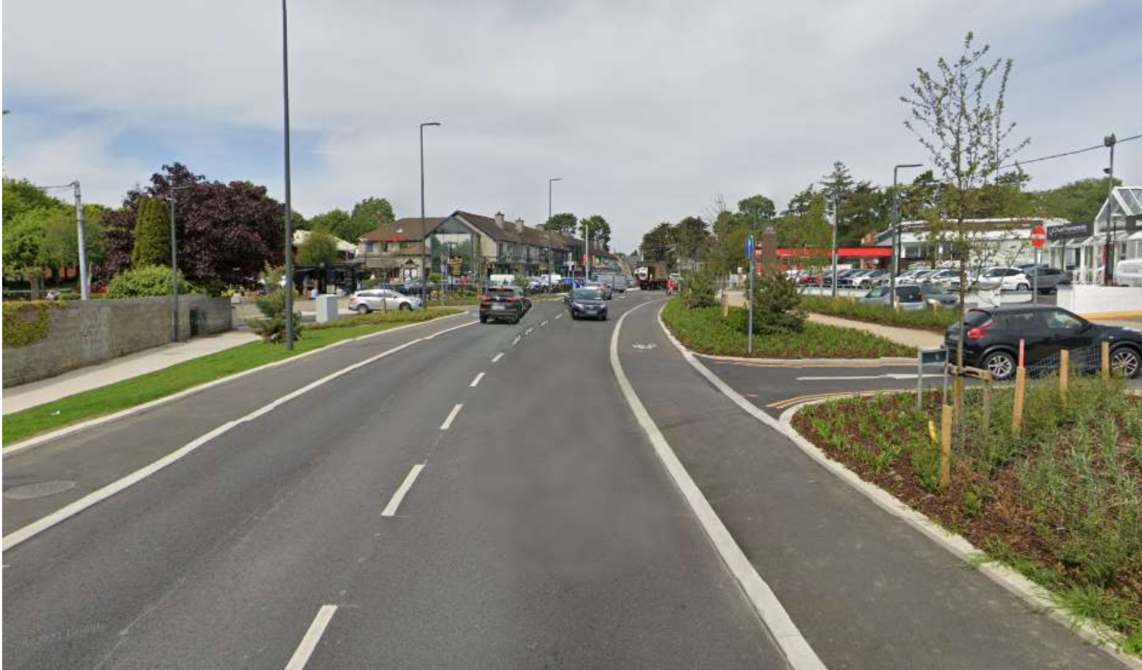
Tightened corner radii at side roads
