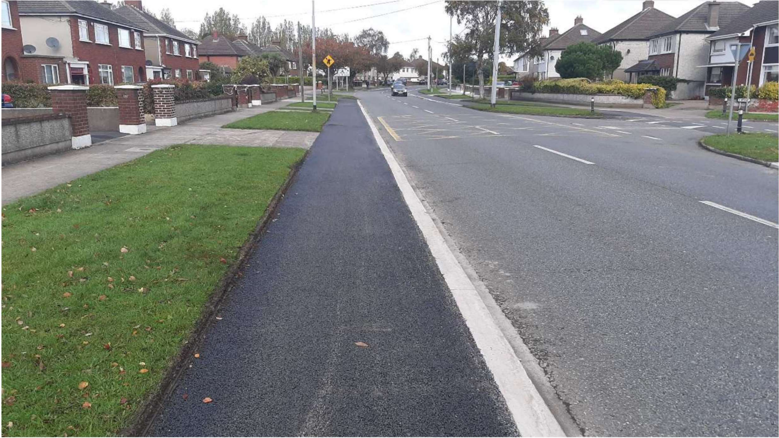
After the upgrade on Cypress Grove Road
