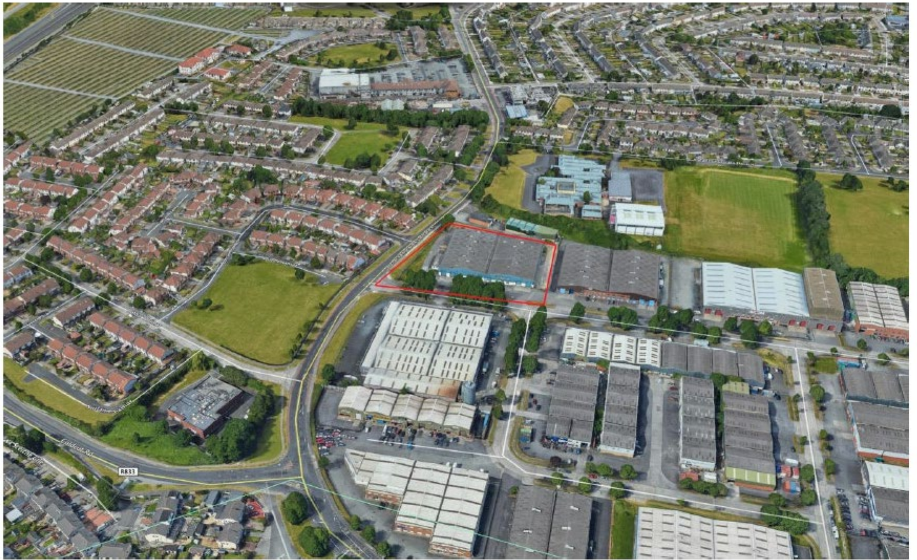
Figure 1.1 – Site and Central Study area looking northwards (Google Earth 3D)
