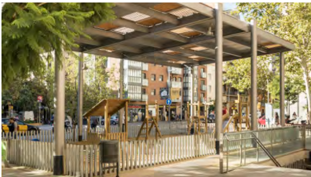
Green by name and green by nature: Integration of eco-friendly approaches, e.g. shelter used for solar energy collection, planting and drainage for rainwater harvesting
