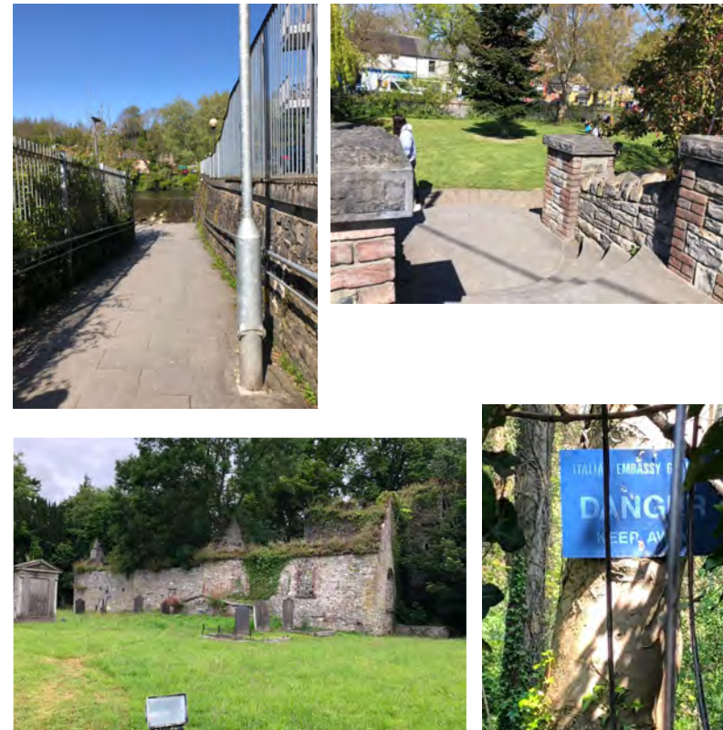
FIG. 3: ILLUSTRATIONS OF AREAS REQUIRING IMPROVEMENT
