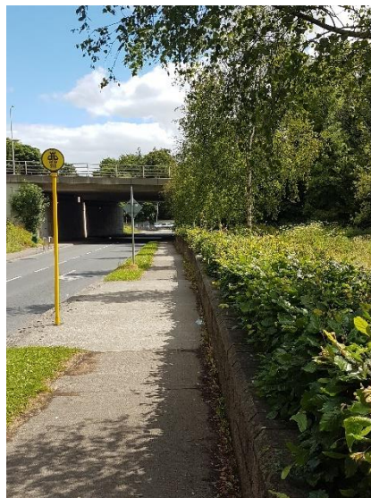
Figure 2-12: Observation – Overhanging Foliage & Tree Growth over Proposed Footway
