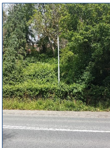
Figure 2-4: Public Lighting Obstructed by Vegetation
