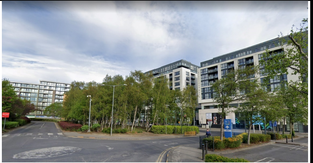
View of Public Realm at Tallaght (The Square) Luas Stop from SE Corner of Site (Google)
