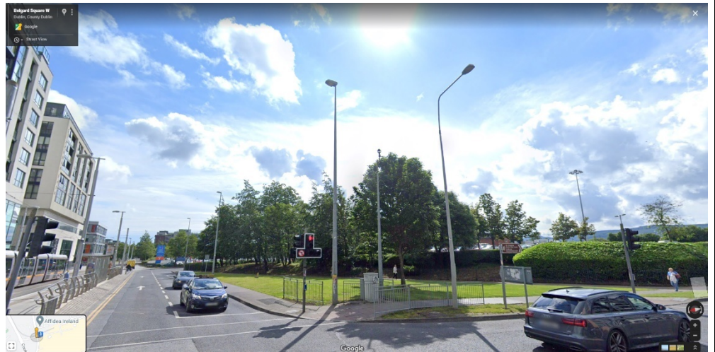
View of Public Realm at Tallaght (The Square) Luas Stop from NW Corner of Site (Google)
