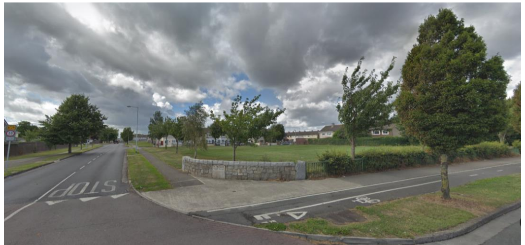
View from the corner of Neilstown Road and St Ronans Avenue (Google)
