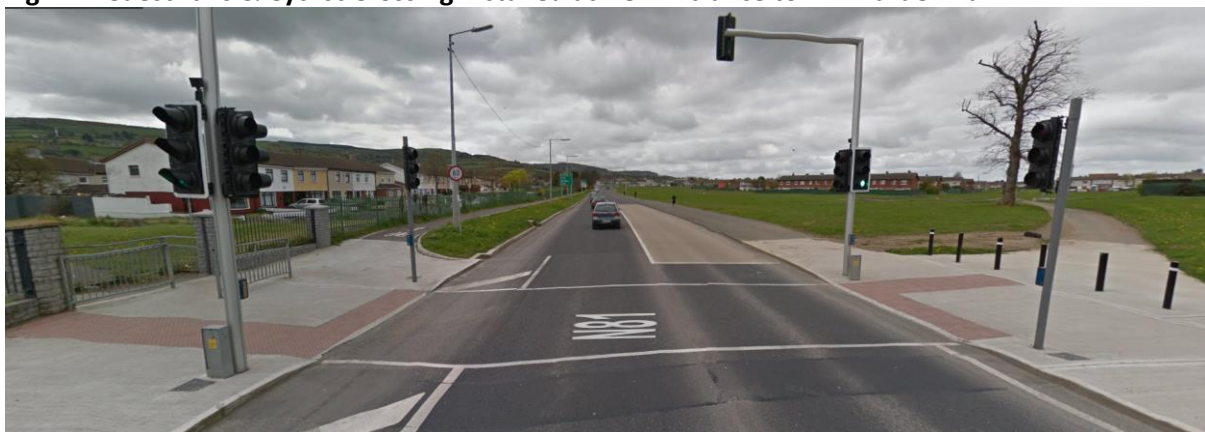
Fig 11. Pedestrians & Cyclist Crossing Installed at N81 Entrance to Killinarden Park
