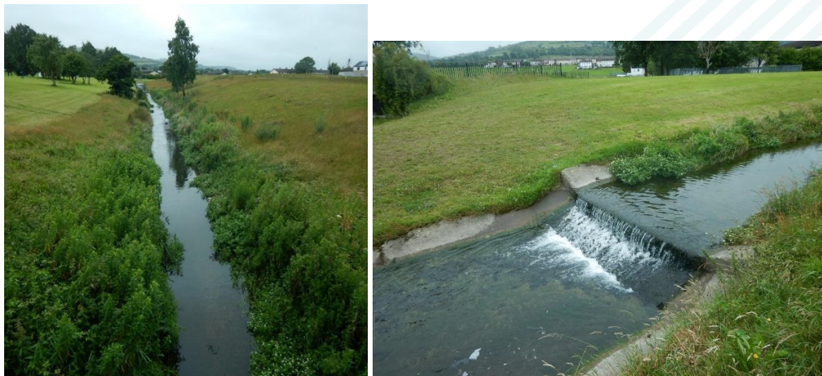
Figure 4-11: Whitestown Stream in Killinarden Park with instream vegetation and concrete weir
