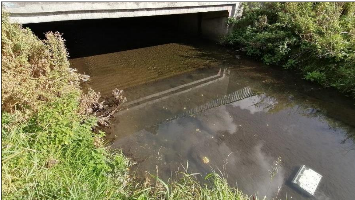
Plate 4.2 An example of rendered concrete bed (i.e. ‘open culvert’) on the Whitestown Stream at site A4, providing very poor instream habitat diversity for aquatica flora and fauna
