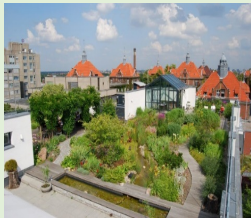
Figure 4.8: Green roof, Berlin.
