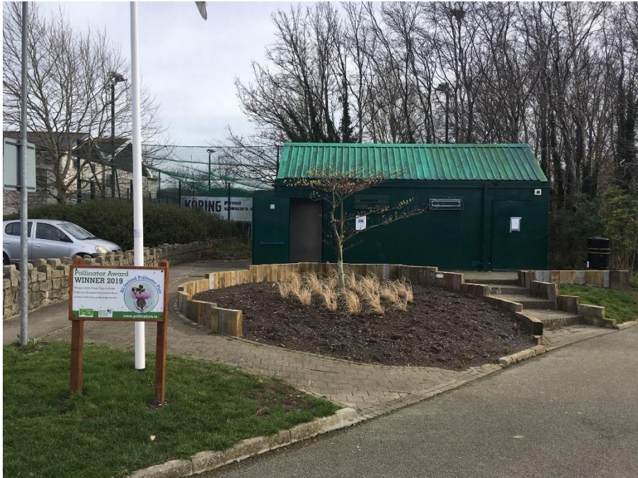
Existing temporary toilet block to be removed to facilitate relocated maintenance entrance
