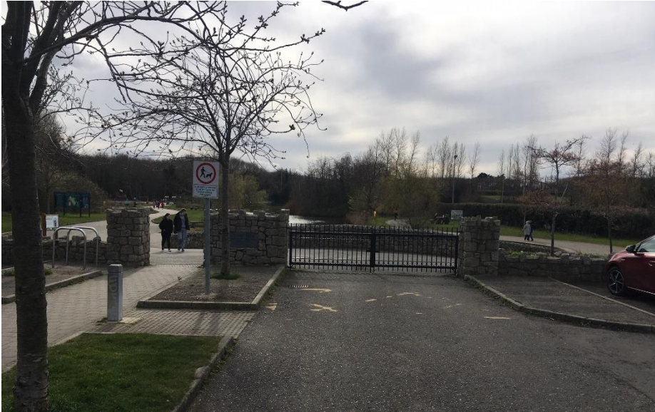
Existing maintenance access to be relocated to south to enhance pedestrian entrance
