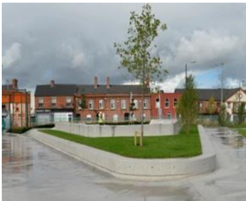
Example of concrete path and concrete kerbs/low concrete walls to contain planting and provide seating
