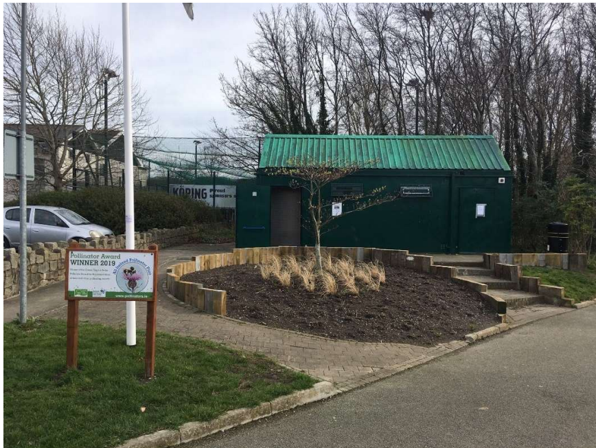
Existing temporary toilet block to be removed to facilitate relocated maintenance entrance
