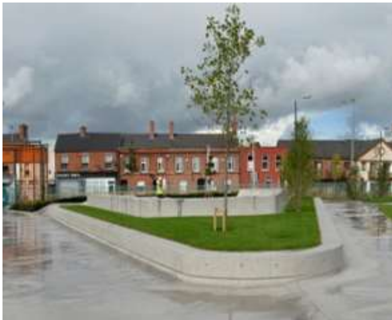
Example of concrete path and concrete kerbs/low concrete walls to contain planting and provide seating
