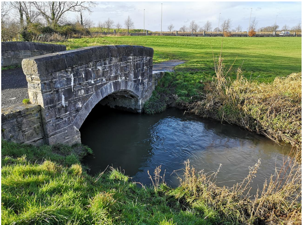
Plate 2 River Camac at bridge to north. Note levels following Storm Ciara
