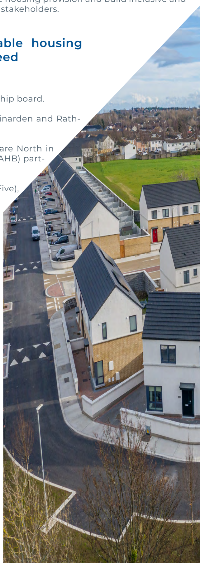
Right: Recently completed housing at St Cuthbert's Meadow, Clondalkin.
