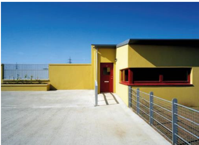
A typical Day-House in Kishogue Park, as existing
