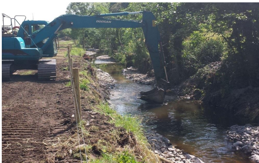
Photo 3: Example of OPW River Enhancements works
