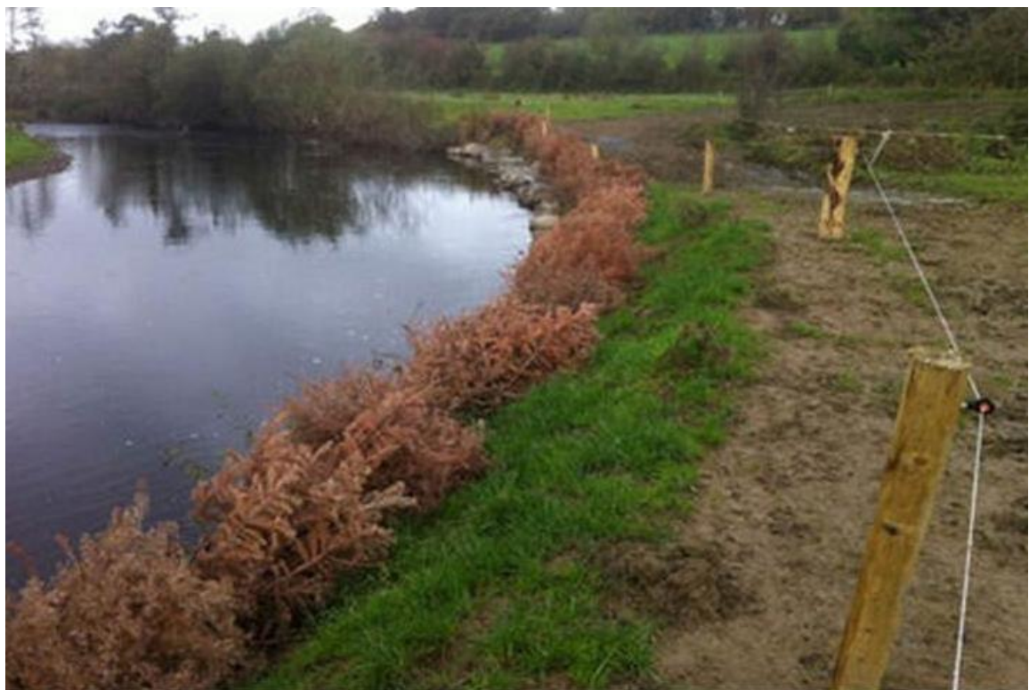
Photo 2: River rehabilitation measure using trees for bank protection (Duhallow IRD 2014).
