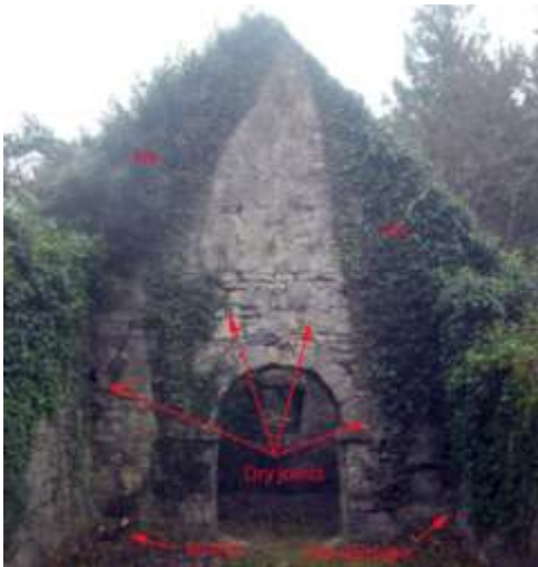
Above: The east face of the chancel arch shows dry joints in the lower half of the wall, while much of the upper half and sides of the arch are concealed by ivy growth.
