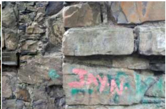
Above: Damaged stone and graffiti (painted & etched) can be seen on the chancel arch.
