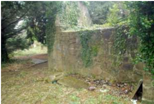
Above: The external face of the north wall of the chancel showing some graffiti, dry joints and vegetation.
