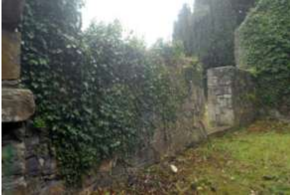
Above: The external face of the south wall of the nave has been previously repaired in OPC-based mortar and shows well-developed ivy, some voids forming in the joints, graffiti and damage to some stones from fires.
