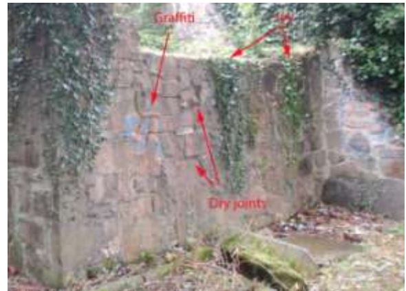
Above: The external face of the north wall of the chancel showing some graffiti, dry joints and vegetation.
