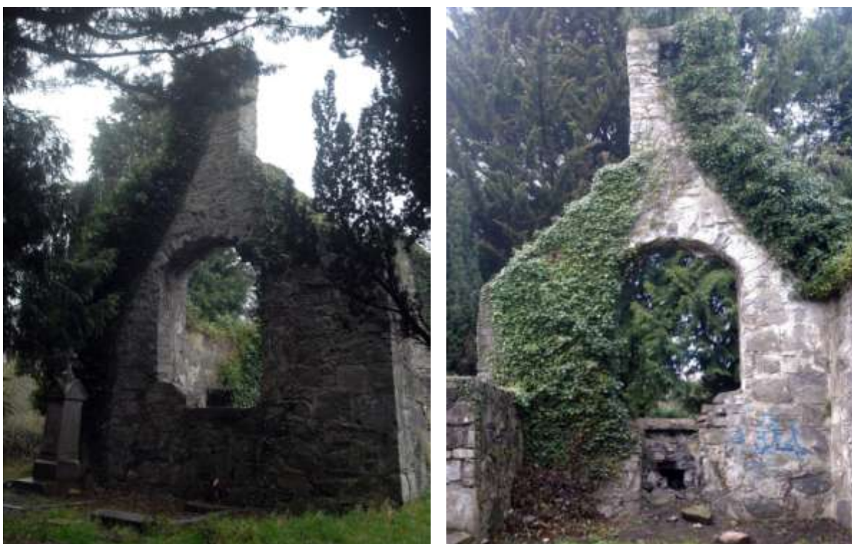
Above: The west gable is overgrown with mature ivy which conceals the southern face of the interior, the northern face of the exterior, and the wall tops. The masonry has been repointed with OPC-based repointing mortar, though original mortars and traces of former external renders and internal plasters survive. The masonry of the blocked-up west doorway has been disrupted, and some graffiti is present on the wall surfaces of the interior.
