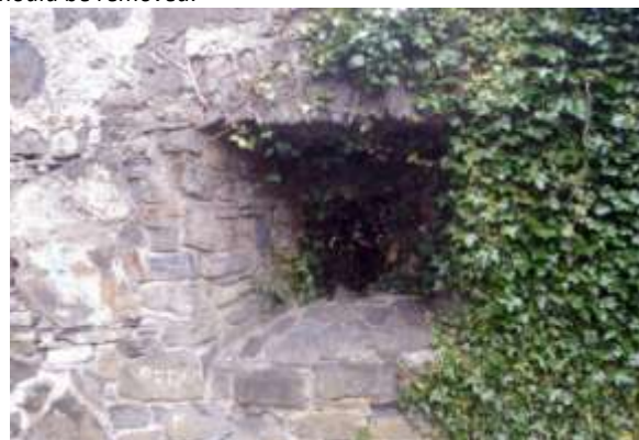
Above: The external face of the east window is obscured by vegetation (left) but the interior (right) appears in good condition though will be similarly obscured without active intervention to control vegetation. Note the survival of plasters on the internal face. Graffiti can also be seen on the exposed stone masonry.
