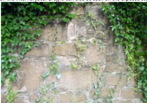
Above: Detail of the masonry exposed on the external face of the north wall. The OPC pointing in this area appears in reasonable condition, though much is obscured by vegetation.
