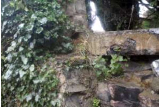
Above: The south side of the doorway is overgrown but the exposed masonry is loose and requires consolidation.
