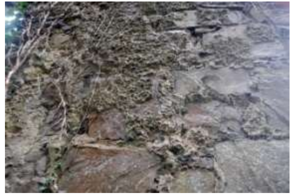
Above: The bellcote (left) shows well-developed vegetation which will begin to disrupt the masonry if left unattended. While vegetation has been removed from the base of the wall, new growth can be seen at the base of the wall and ivy can also continue to grow higher up on the wall where the root systems have established a foothold. The external and internal surfaces of the wall also retain traces of original renders and lime pointing (right) which should be retained.
