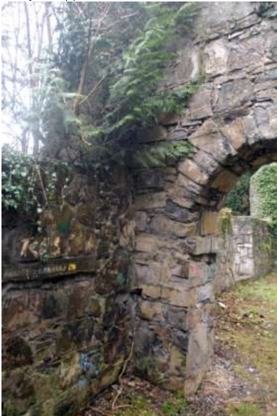
Above: The east face of the chancel arch repeats the pattern seen on the west face – with a need for removal of the ivy growth and local pointing-up of dry joints.
