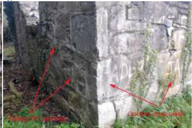
Above: The south-west corner of the masonry contains some cracked stone suggesting minor movement of the structure. OPC joints have also failed in this area.
