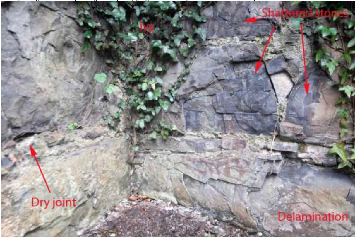
Above: Degradation of the masonry arises from the development of ivy, the burning of fires which is damaging the stones, and loss of mortar from the joints (which destabilises the masonry).
