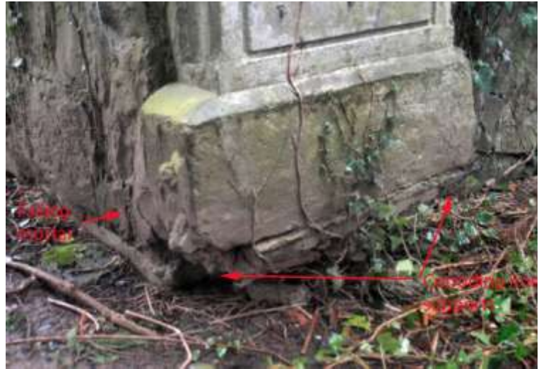
Above: The memorial attached to the south-east corner is held by corroding iron supports.
