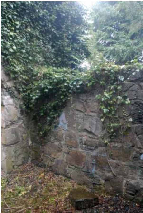
Above: The internal face of the north chancel wall appears in reasonable condition. However, the vegetation may conceal some minor failures.
