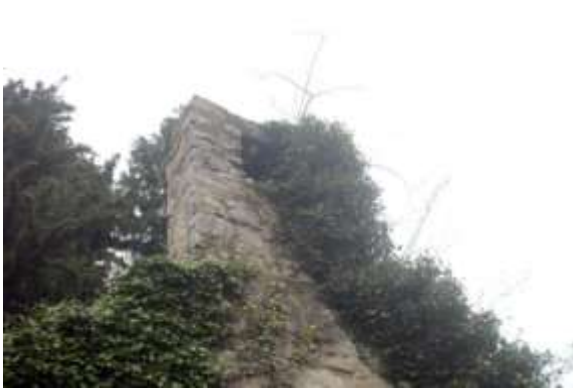
Above: The bellcote (left) shows well-developed vegetation which will begin to disrupt the masonry if left unattended. While vegetation has been removed from the base of the wall, new growth can be seen at the base of the wall and ivy can also continue to grow higher up on the wall where the root systems have established a foothold. The external and internal surfaces of the wall also retain traces of original renders and lime pointing (right) which should be retained.
