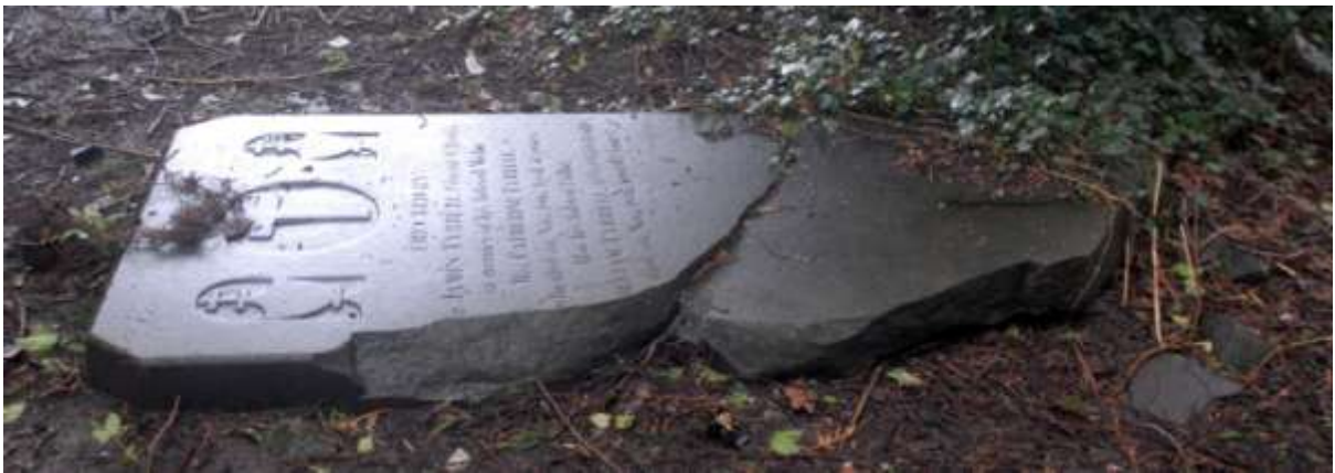
Above: This stone has been badly damaged. These types of cracks are spalls are most likely to arise from impact damage.
