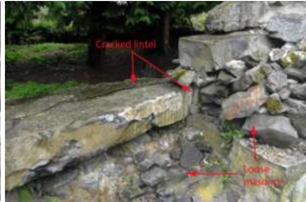
Above: The surviving half-lintel has cracked along its length and also cracked where it meets the jamb. It should be noted that any further vandalism with this lintel will result in its collapse. The surrounding masonry is loose and requires consolidation.
