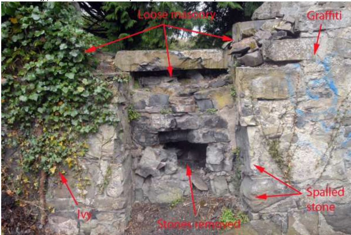
The internal face of the west doorway is in very poor condition. The blocked-up work has been interfered with and no longer adequately supports the lintel. The lintel and adjacent masonry is loose and liable to collapse. In comparison, the graffiti, while
