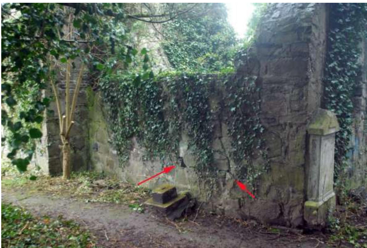
Above: Vertical structural cracks (arrowed in red) illustrate an area at risk of collapse.
