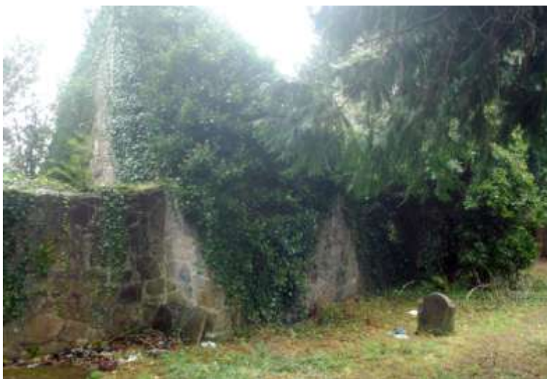
Above: The condition of the external face of the north wall of the nave is largely concealed behind vegetation. A tree is growing in close proximity to the window (above right). This tree should be removed.
