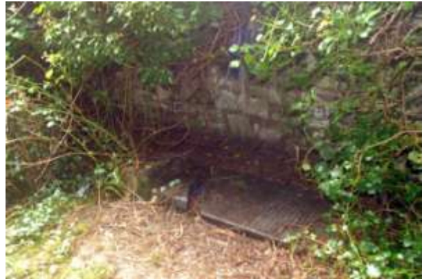
Above: This cracked memorial lies adjacent to the boundary wall and appears to be somewhat protected from anti-social behaviour within the graveyard. It is possible to re-erect and secure cracked slabs such as this once the church building has been secured.
