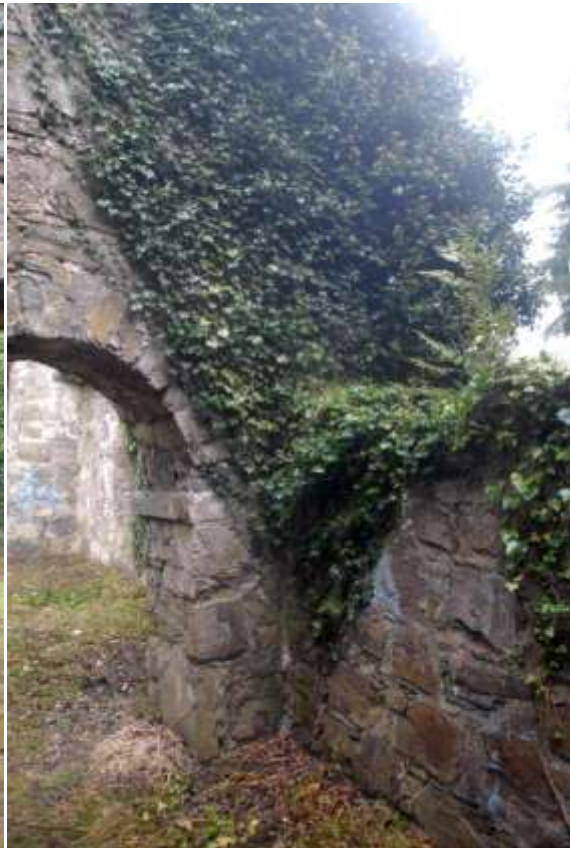
Above: The east face of the chancel arch repeats the pattern seen on the west face – with a need for removal of the ivy growth and local pointing-up of dry joints.
