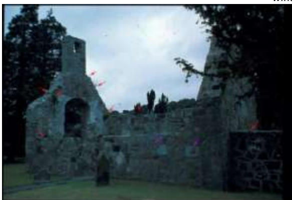
Above: Photo of the church by Patrick Healy noted c.1992 11 , showing plant growth in joints and/or horizontal surfaces (arrowed in red) and graffiti (arrowed in purple).
