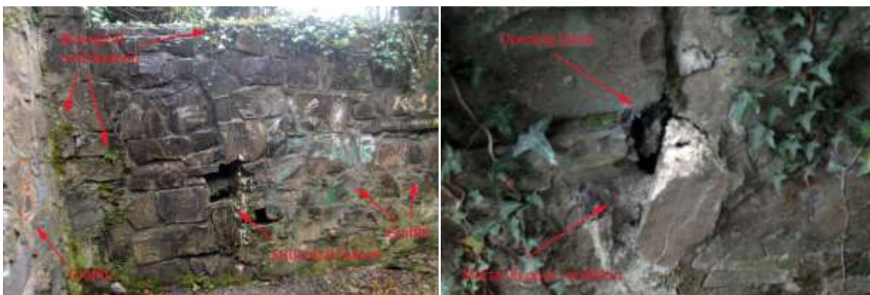
Above: The corresponding internal face of the wall shows voids in the masonry corresponding with the structural cracks visible externally, and plant growth in the joints indicating both mortar failure and saturated masonry. Vegetation has also colonised the walltops and graffiti can be seen on the internal face of the chancel.
