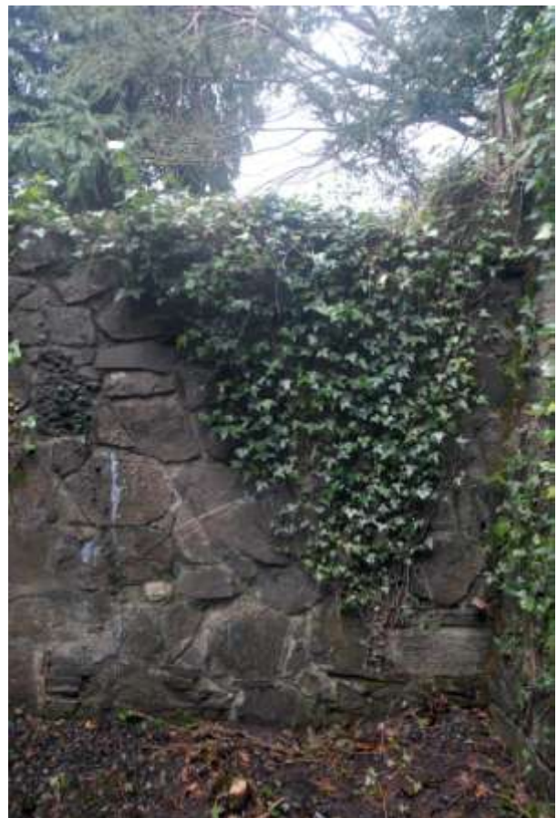
Above: The internal face of the north chancel wall appears in reasonable condition. However, the vegetation may conceal some minor failures.
