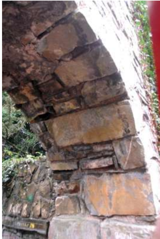
Above: The intrados of the chancel arch shows some dry joints (mainly on the south side) and retains evidence that it was formerly plastered.
