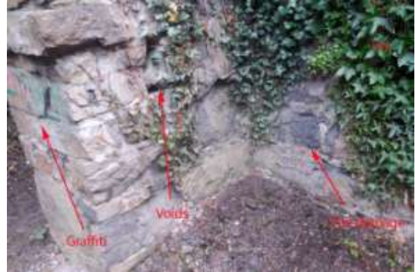
Above: The external face of the south wall of the nave has been previously repaired in OPC-based mortar and shows well-developed ivy, some voids forming in the joints, graffiti and damage to some stones from fires.
