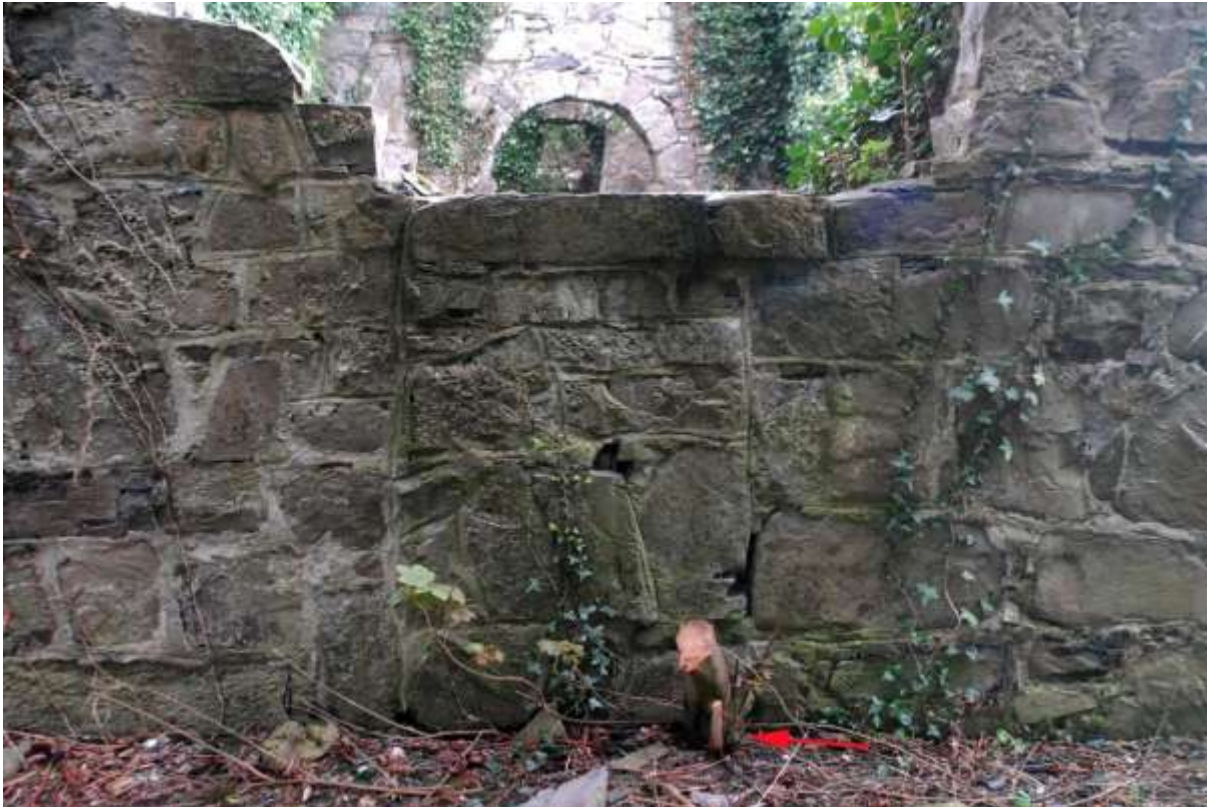
Above: The west door is generally considered to be early (sloping jambs and a flat lintel). The distinctive jambs stones illustrated by Wakeman in 1892 (see Section 2.2) have been obscured by OPC repointing and the lintel has cracked and dropped. These OPC mortars are in poor condition and have lost bond with the limestone masonry in many locations, with open dry joints visible within the blocked-up work. Ivy growth is re-generating and should be removed. A young tree/shrub has been cut off (arrowed) but this is also likely to re-generate and the stump should also be removed.
