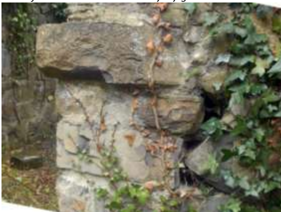
Above: Deep dry joints are evident in the masonry surrounding the chancel arch.
