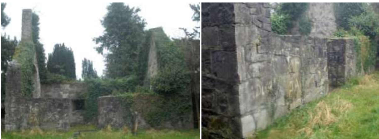
Above: The south wall of the nave has been capped and repointed with OPC mortars. The external wall face shows well-developed vegetation cover, particularly at the east end but with new growth developing at the west end also. Graffiti is also present.
