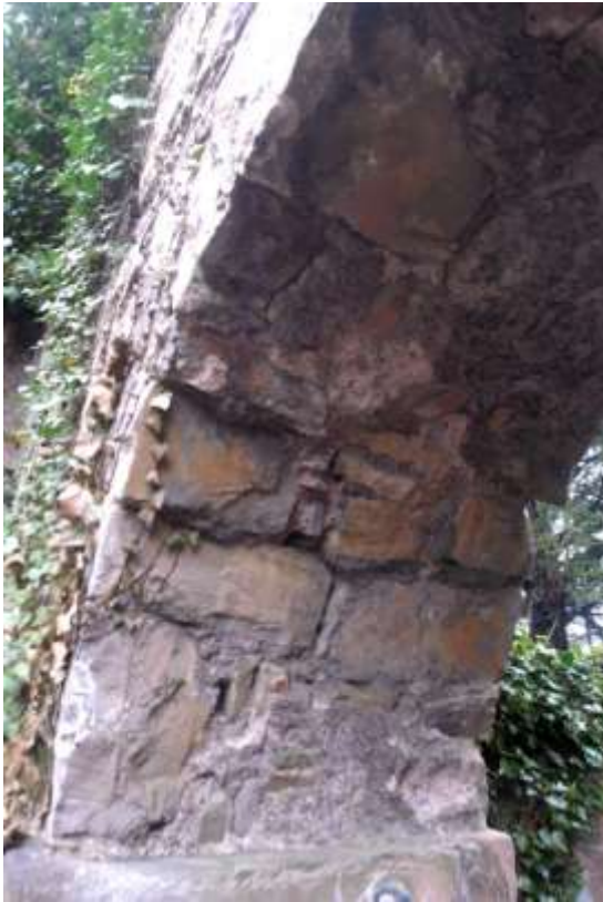
Above: The intrados of the chancel arch shows some dry joints (mainly on the south side) and retains evidence that it was formerly plastered.
