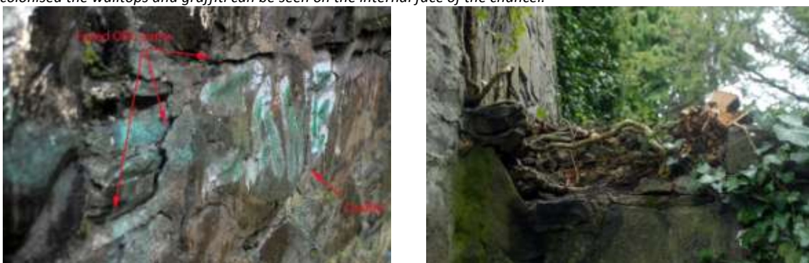
Above: The graffiti while unsightly is not as damaging to the fabric of the church as the failing mortar joints (left) while the vegetation on the walltops conceals disruption of the tops of the walls (right).
