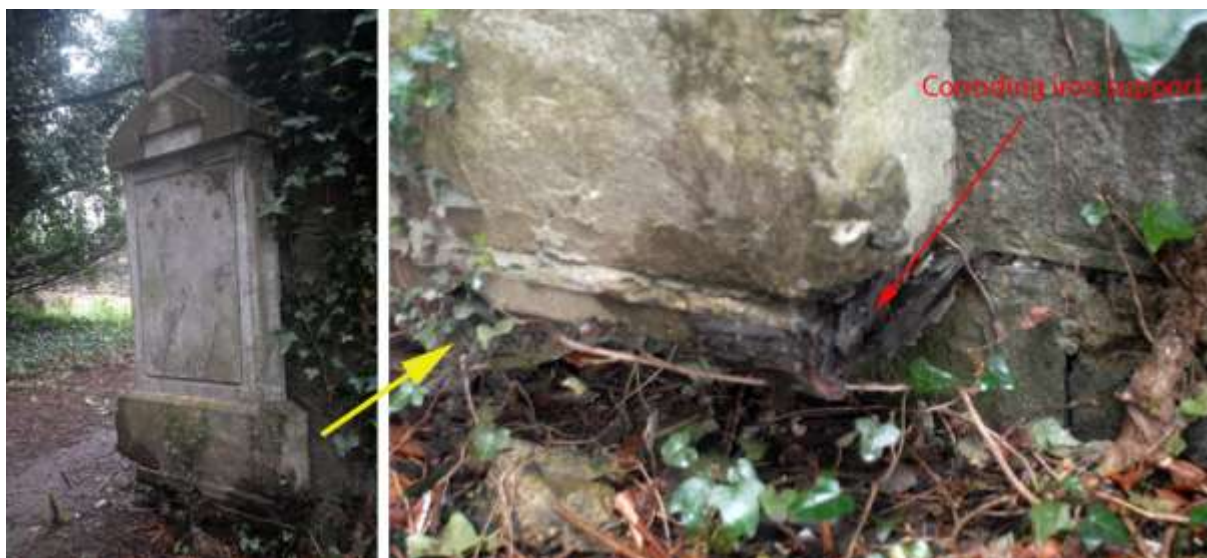
Above: This memorial attached to the south-east corner of the chancel is vulnerable to collapse, but very small works to treat the iron and consolidate the base would ensure its survival.
