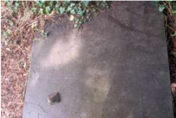
Above: The lettering on this graveslab has become difficult to read as the surface of the stone weathers back. The surface has suffered from graffiti (etching) which has permanently damaged the surface.
