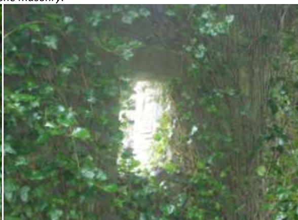
Above: The north window is heavily obscured, however the masonry appears in reasonable condition and it should be possible to carefully remove the ivy and other plant growth without significant damage to the masonry.
