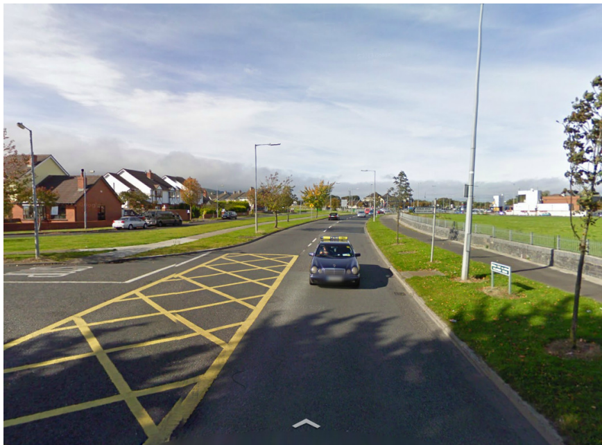
View on Killinniny Road at Old Court Rd junction showing future site access
