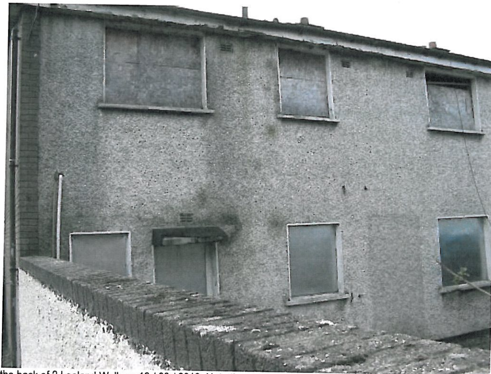
A view of the back of 2 Lealand Walk on 13 / 03 / 2013. Note the stains and dampness on the wall, the cable and the breach in the plywood sheet which secures one window opening at first floor level.
